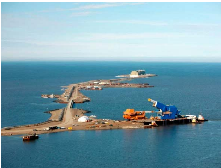
Figure 4.1-2. Parker Drill Rig Offloading at West Dock 2, Prudhoe Bay
