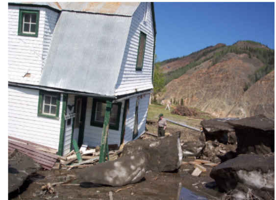
Eagle Custom House after 2009 flood
