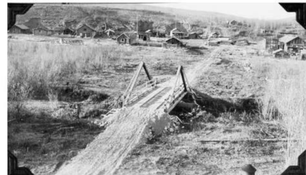
Bridge crossing Livengood Creek in Livengood, c. 1938.
