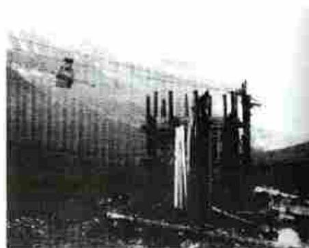
Image E-16 Tramway on a Trestle Leading from the Rock Crusher to the Mill at Sealevel Mine (Source: Mining and Scientific Press (newspaper), San Francisco, May 9, 1903)
