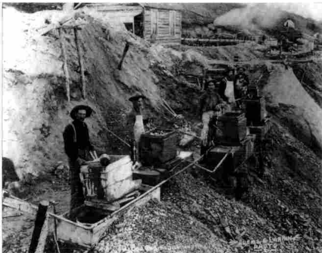
Image E-3 Rockers Used to Wash Gravel (Yukon Archives 3298)
