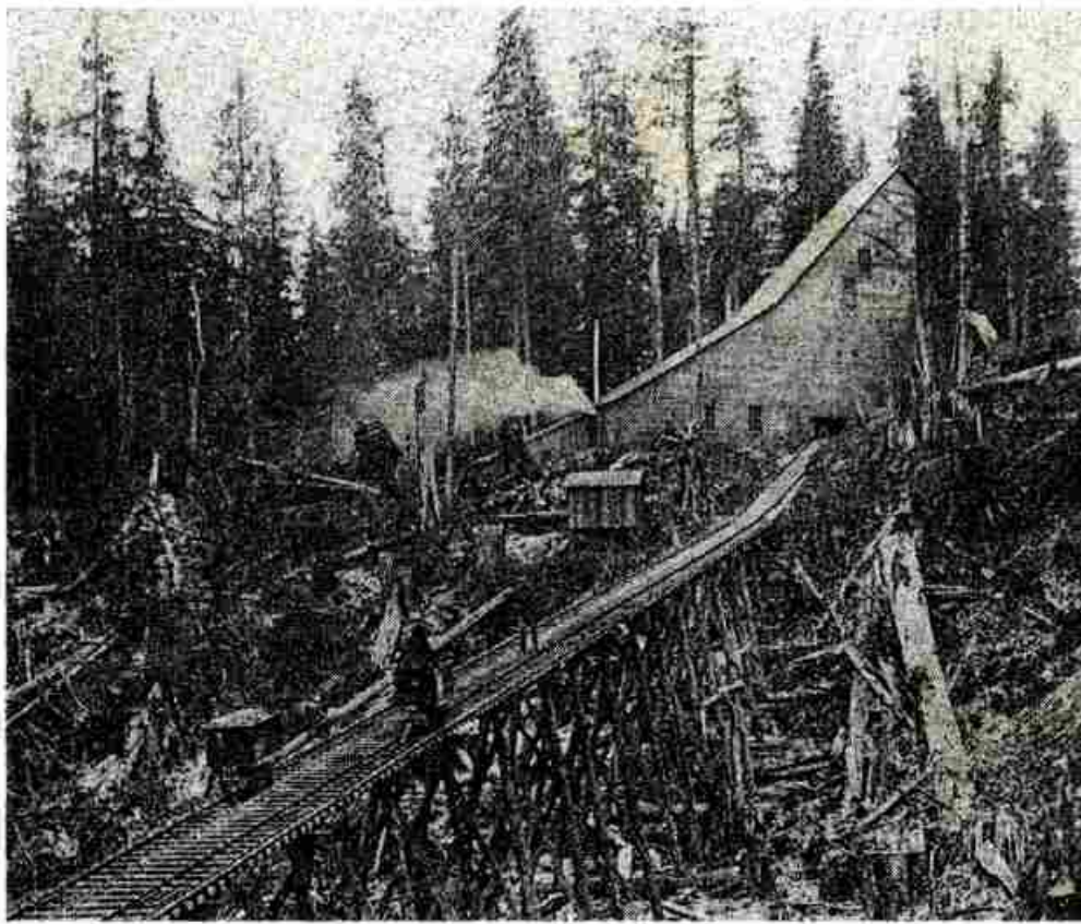
Image E-16 Tramway on a Trestle Leading from the Rock Crusher to the Mill at Sealevel Mine (Source: Mining and Scientific Press (newspaper), San Francisco, May 9, 1903)
