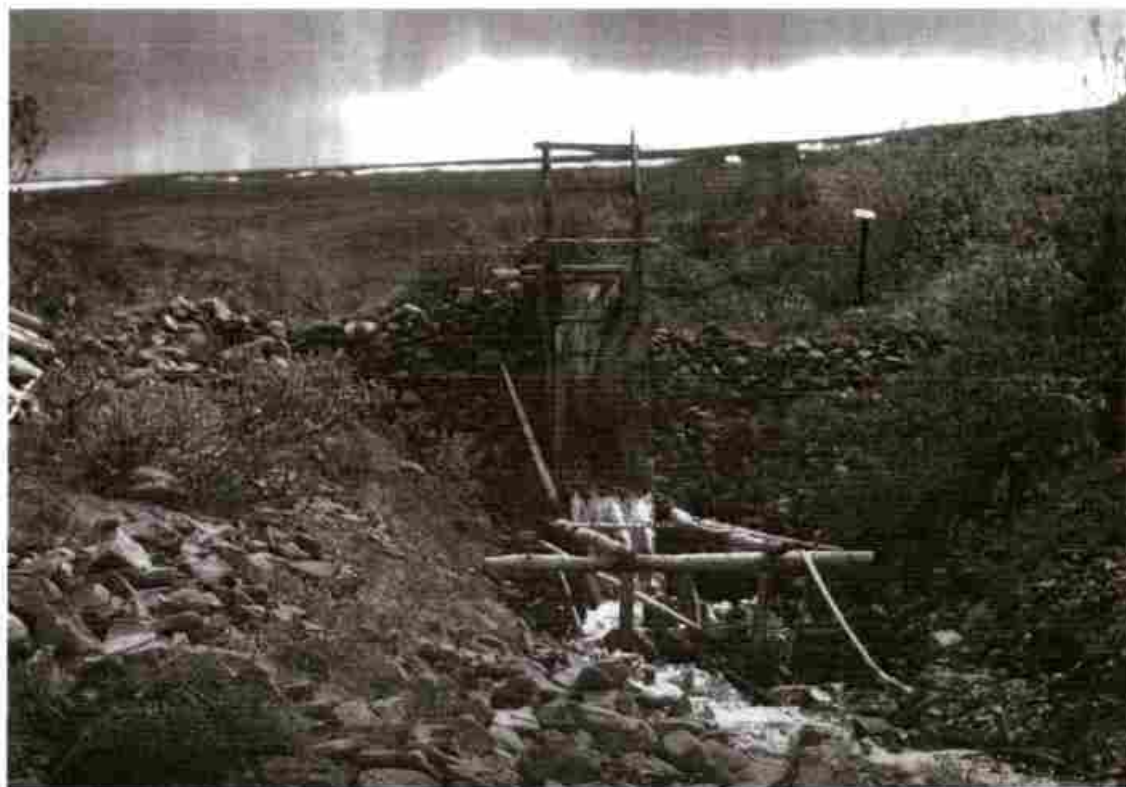
Image E-8 Boomer Dam Used in Ground-Sluicing at Gold Run Creek (Source: Becky M. Saleeby, The Quest for Gold , National Park Service, 2000)
