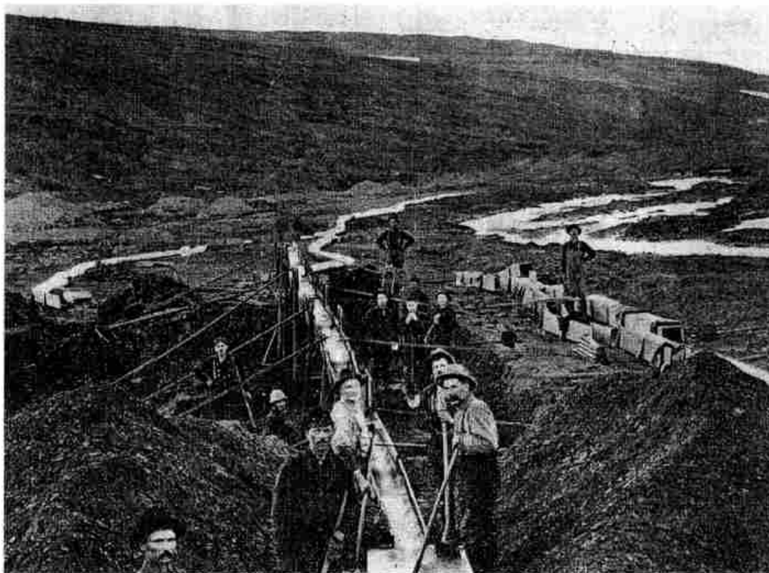
Image E-5 Shoveling Rock into a Sluice at Anvil Creek (Source: Mining and Scientific Press (newspaper), San Francisco, January 9, 1909)
