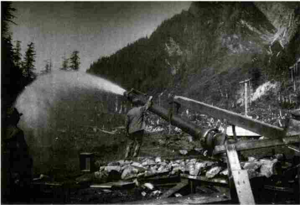
Image E-9 Hydraulic Surface Mining at the Last Chance Mine (A.H. Brooks Collection 572 U.S Geological Survey) (Source: Becky M. Saleeby, The Quest for Gold , National Park Service, 2000)
