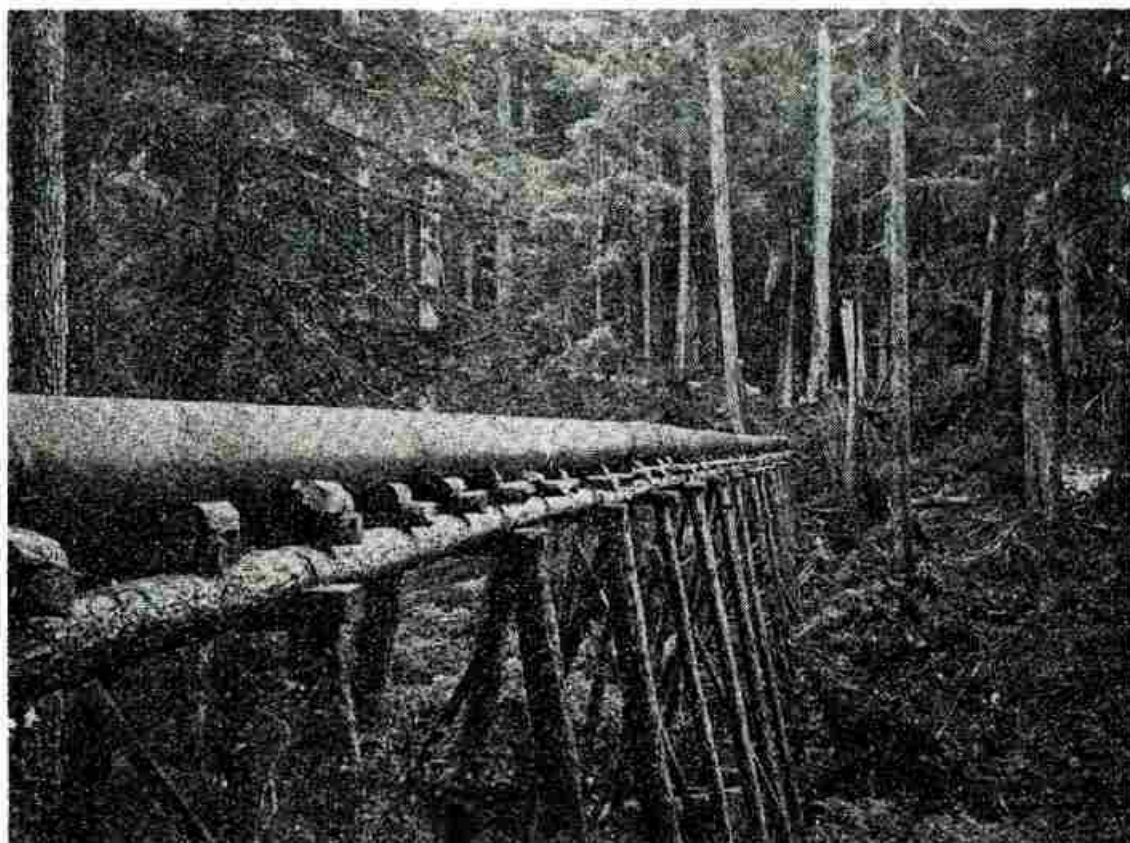
Image E-21 Trestle Supporting Aqueduct Transporting Water to the Mill at Sealevel Mine (Source: Mining and Scientific Press (newspaper), San Francisco, May 9, 1903)
