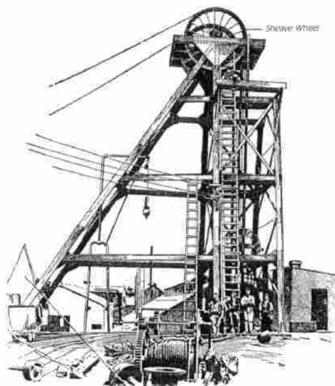
Image E-14 Headframe Used to Transport Personnel and Equipment in a Mine Shaft (International Correspondence School Reference Library, volume 148) (Source: Beth and Bill Sagstetter, The Mining Camps Speak , Benchmark Publishing of Colorado, Denver, 1998)
