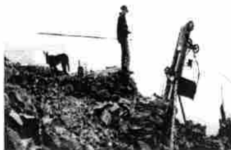
Image E-17 Aerial Trams to Transport Rock from the Mine to the Mill at Yellow Band Mine (photo courtesy of Sylvia Baldwin) (Source: Paul J. White, Cultural Landscape Report, Bremner Historic District , Michigan Technological University for National Park Service, 2000)
