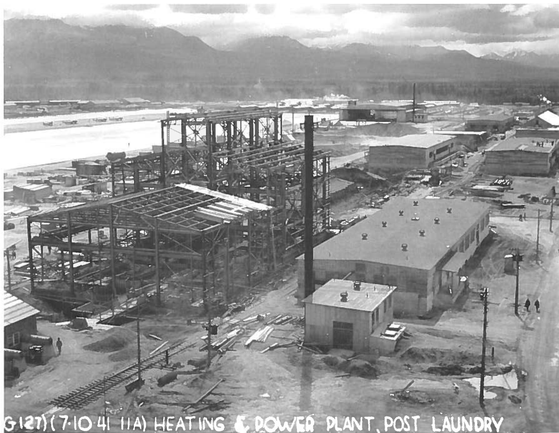
Figure 18. Construction of the Heating and Power Plant (now destroyed) and Building 11-420, the Laundry Facility.
