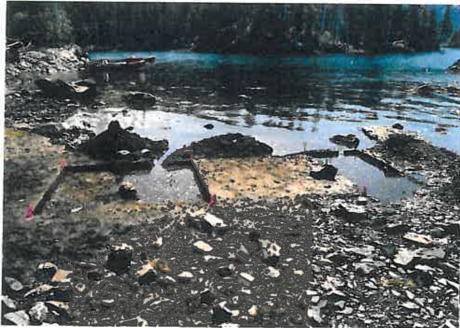
Figure 9: SEL-215, trench flooding by incoming tide.
