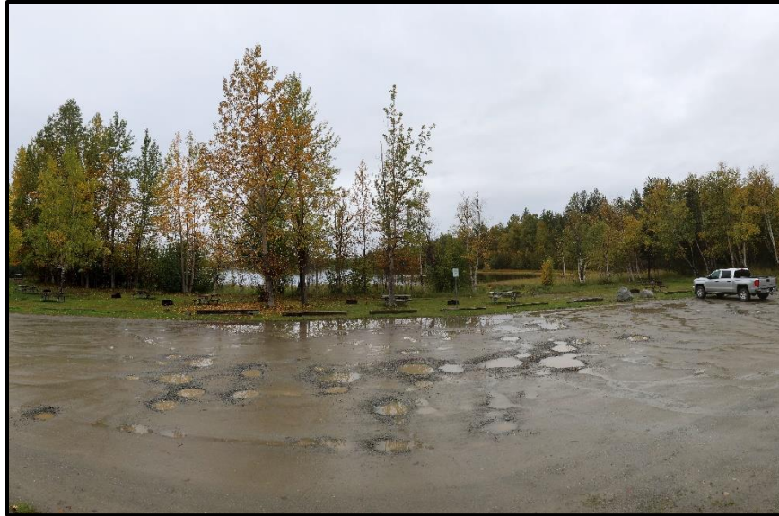
Figure 3 - Potholes at the Boat Launch Parking Area
