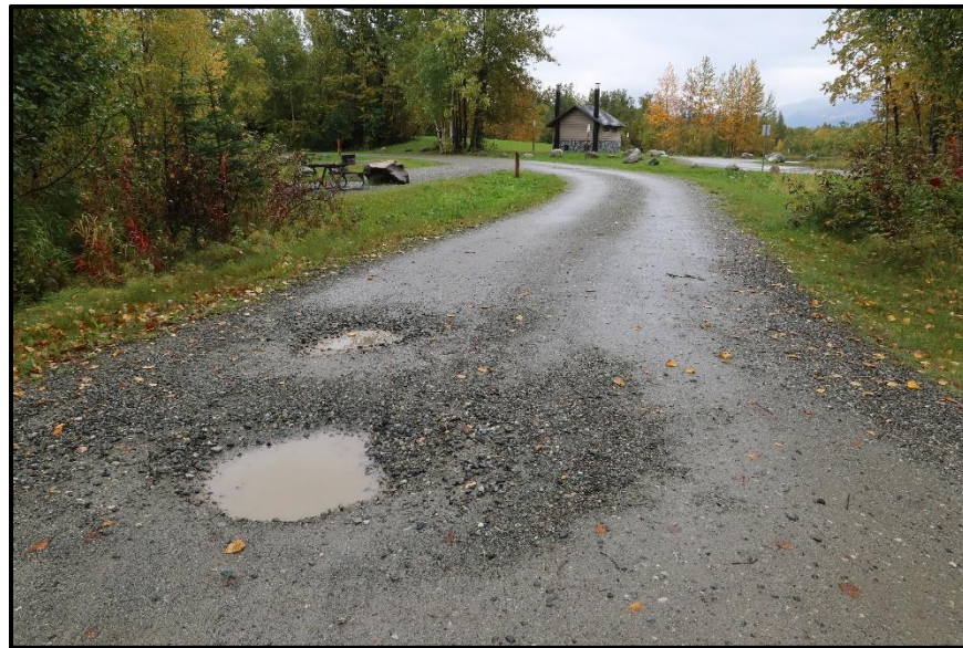
Figure 2 - Potholes Along the RV Campground Road
