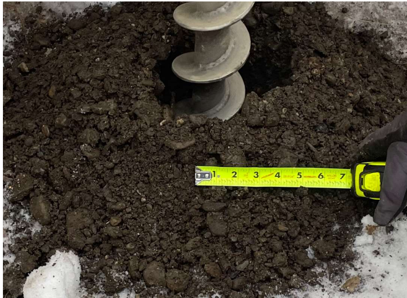
Figure 1: BH-1 Bottom of boring material.
