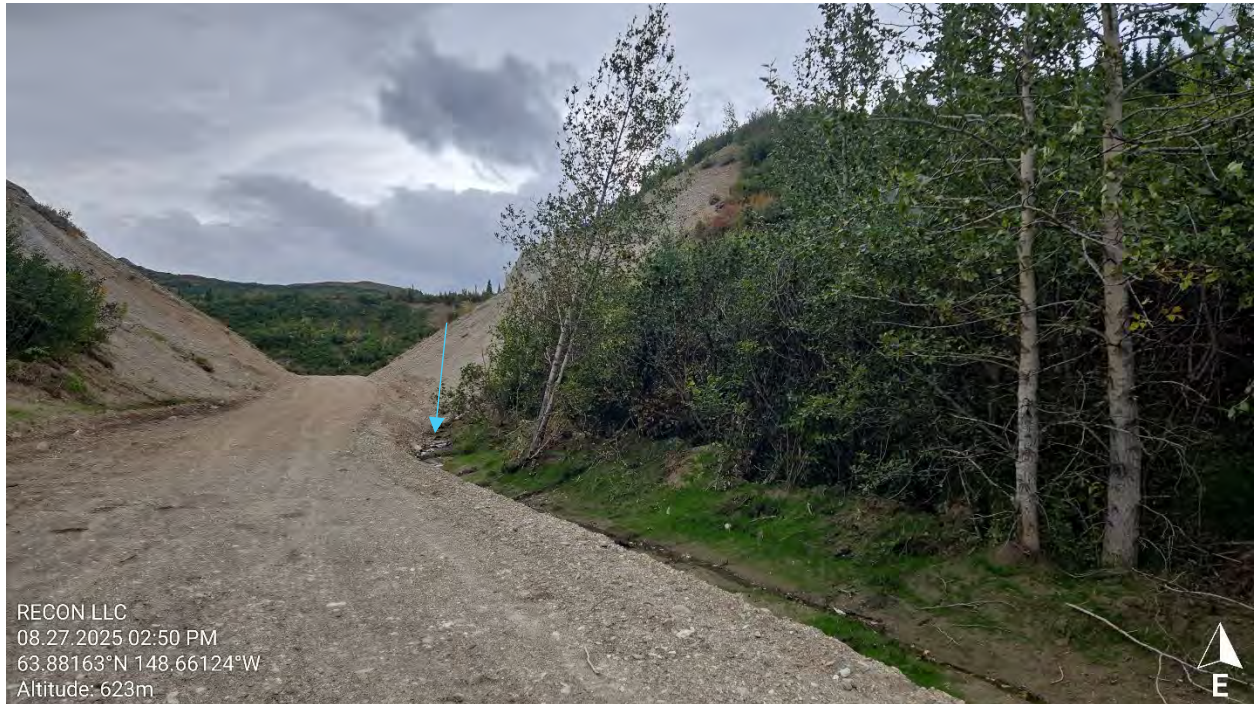
Figure 7: Seep (indicated by blue arrow) west of re-established access road to bottom of Center Pit (view south).
