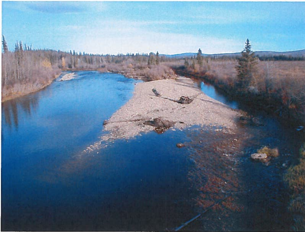
Fig. 4. Downstream of the bridge, the channel is wider, shallower, and has more obstructions from islands and boulders (rock gardens), than upstream of the bridge
