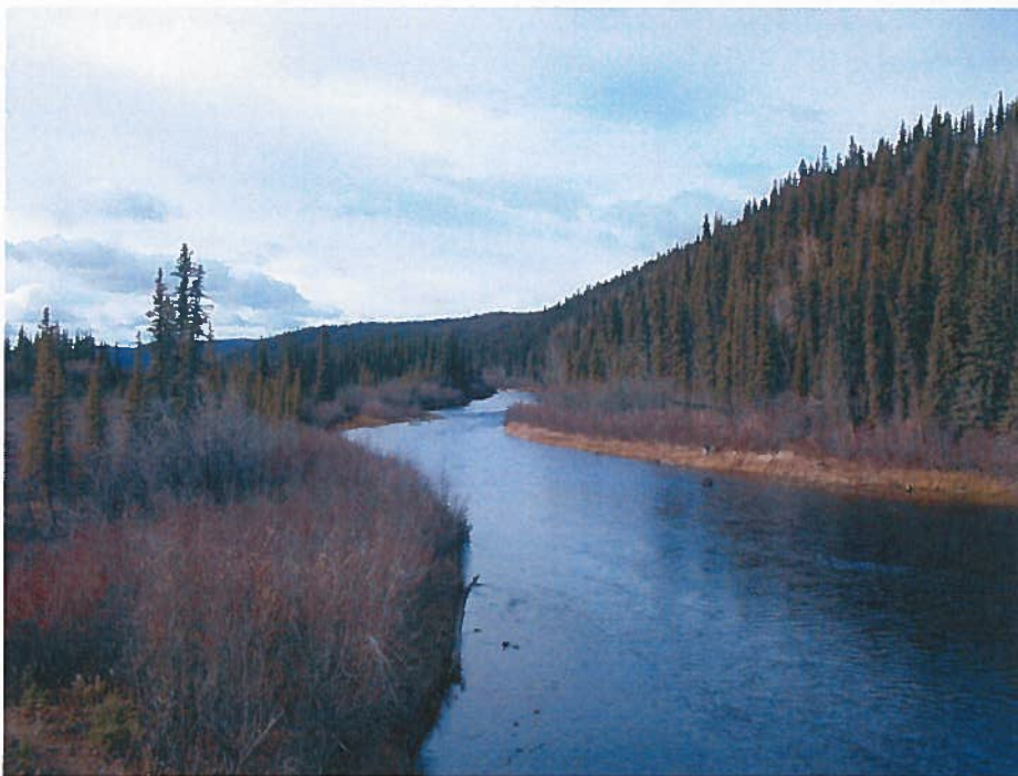
Fig. 3. The channel is relatively straight upstream of the bridge with few riffles or obstructions. The stream is confined by a low ridge to the north with a lower bank and wide floodplain to the south
