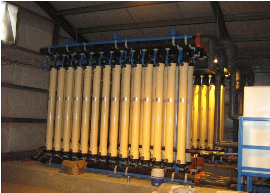
One of two micro-filtration skids
