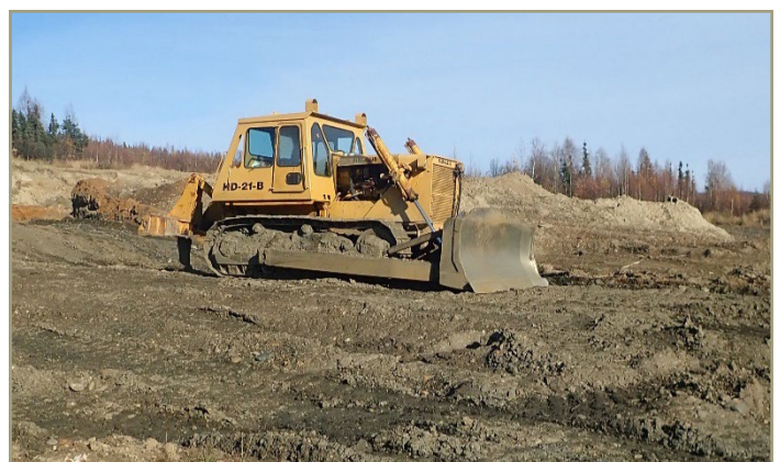
Photo 16. Dozer, Hot Springs Mining District Alaska 2021 (DNR).
