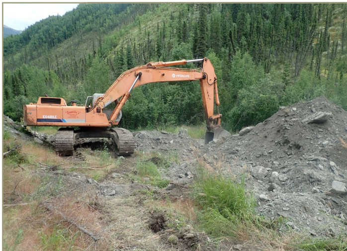
Photo 11. Placer trench exploration in the Rampart Mining District (DNR).
