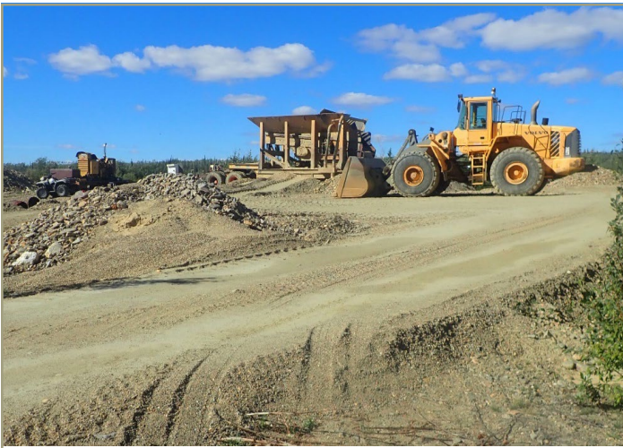
Photo 18. Loader, Central Mining District Alaska 2022 (DNR).
