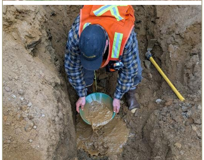
Photo 12 (a), (b) and (c). Photo 12 (a). Preparing to dig out a measured and marked test pit/trench. Photo 12 (b). Removing a grab sample from a potential pay layer in a hillside. Photo 12 (c). Panning a gravel sample in pay layer at the bottom of a test pit (BLM).
