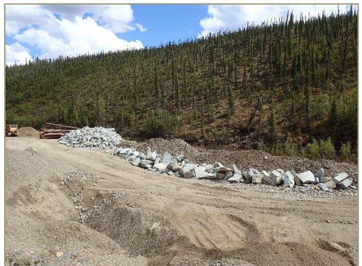
Photo 34. Additional material to stockpile includes boulders, large cobble, and logs, which can be used for stream and floodplain reclamation. From BLM’s “Stream Reclamation Basics.”
