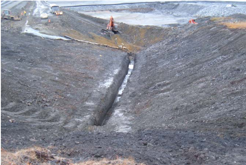
Cutoff Trench and Excavation for Cutoff Wall Extension
