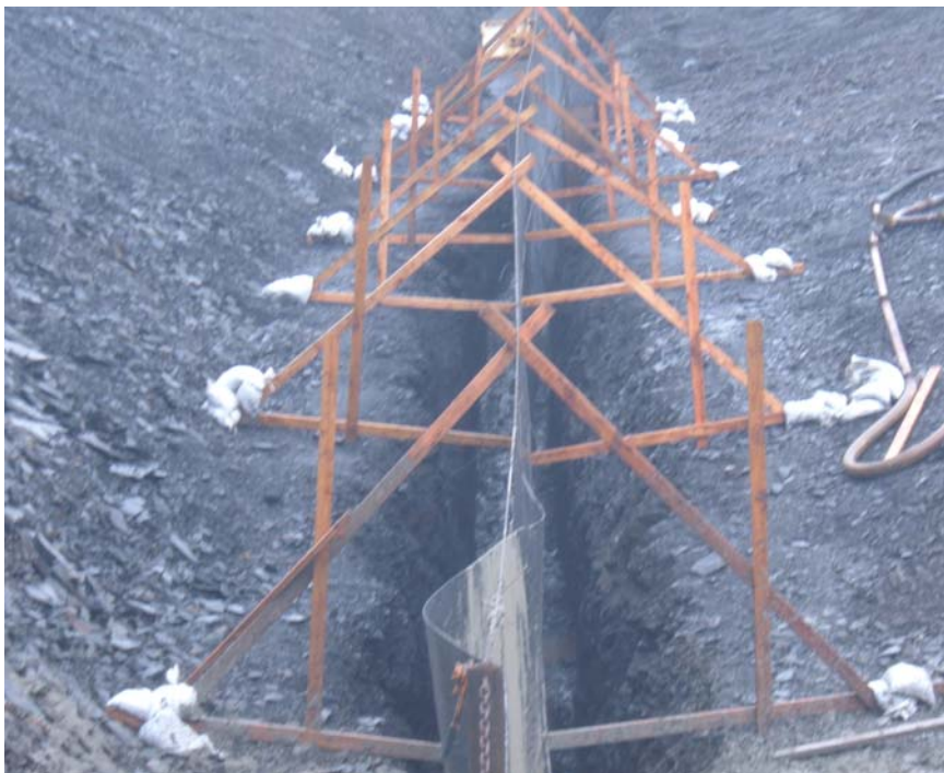
Cutoff Wall Excavation & Geomembrane
