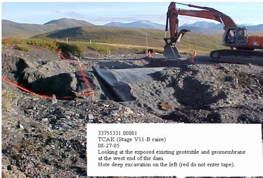
Exposed Stage VII-A Geomembrane at West Abutment
