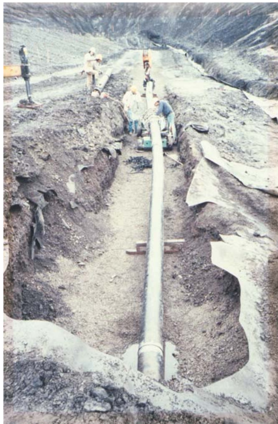
12-Perforated Pipe Toe Drain in Cutoff Trench to Intercept Seepage
