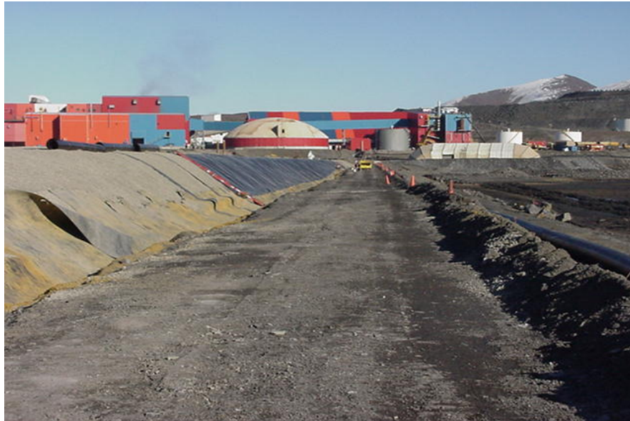
Bedding, Geomembrane, Cover & Buttress
