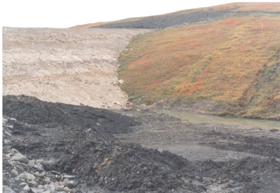
Edge of random rock fill looking towards starter dam. Very soft material approximately 6 to 7 feet thick.
