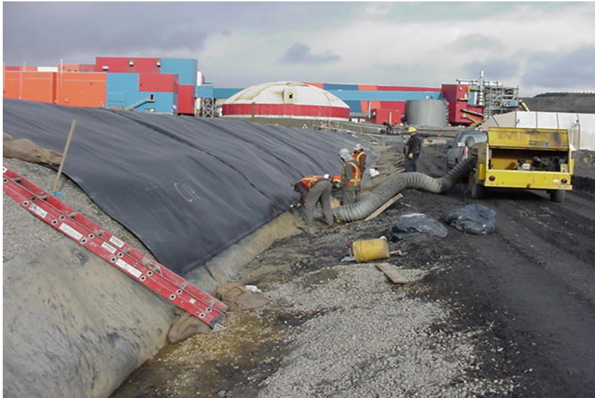
Geomembrane Panel Seam Welding
