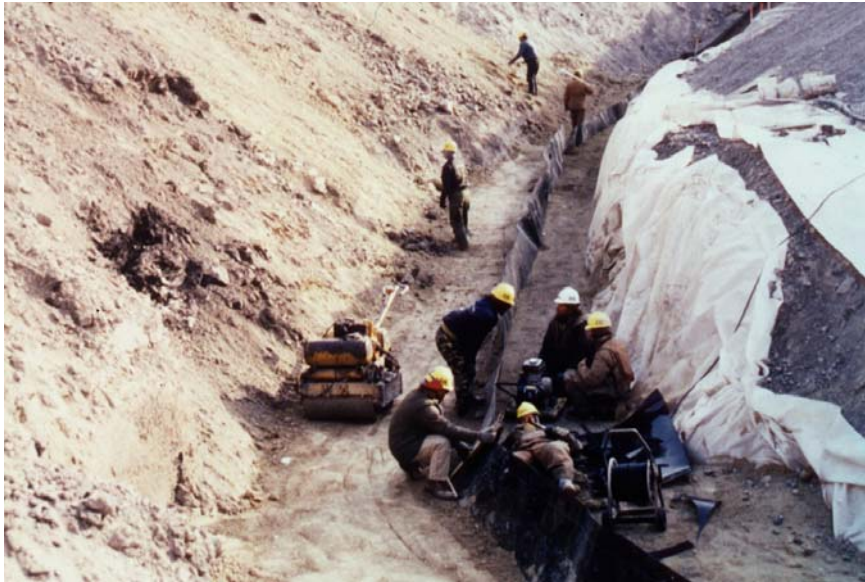
Cutoff Trench to Bedrock at Upstream Toe of Dam
