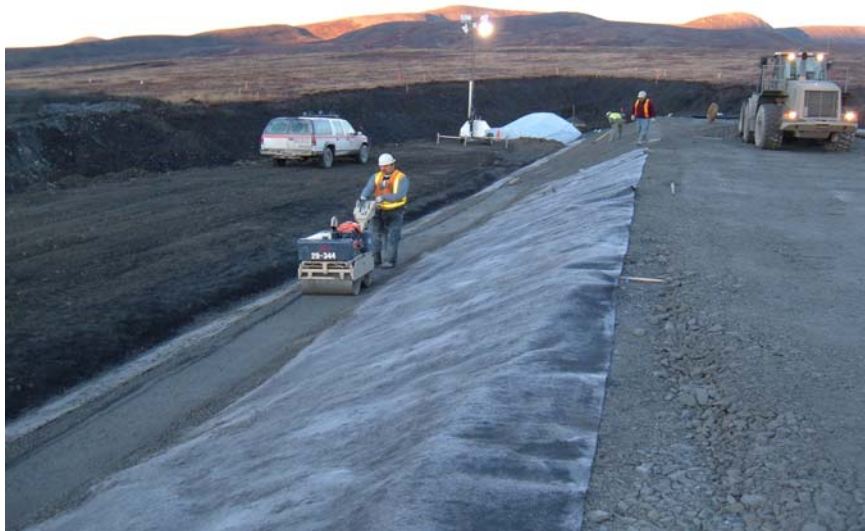
Compacting Liner Bedding on Type II Geotextile
