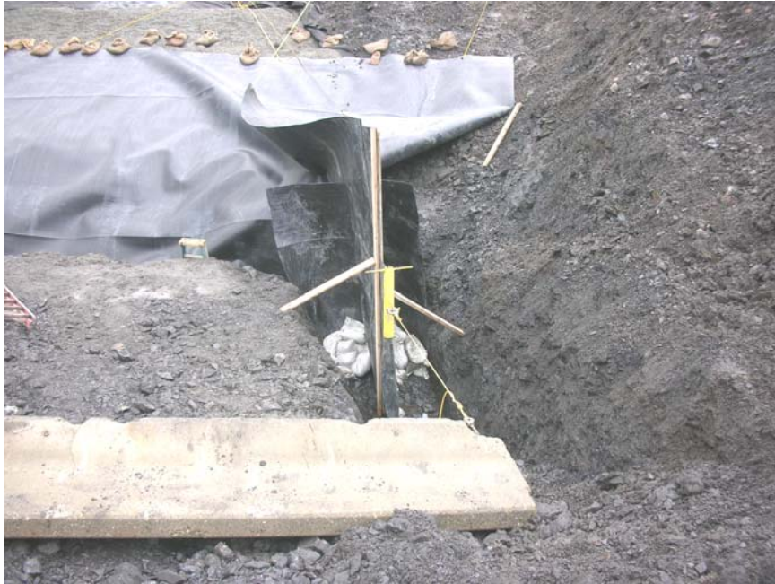
Cutoff Wall to Curtain Wall Transition
