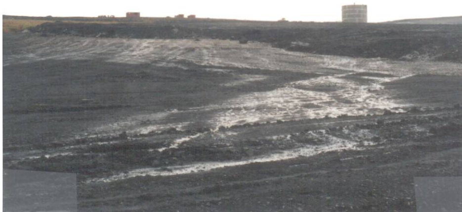
Taken from the seepage dam access road looking towards the east. Lift is estimated to be approximately 5 to 6 feet thick in the middle and tapered on the edges. Noticeable drainage from under lift.
