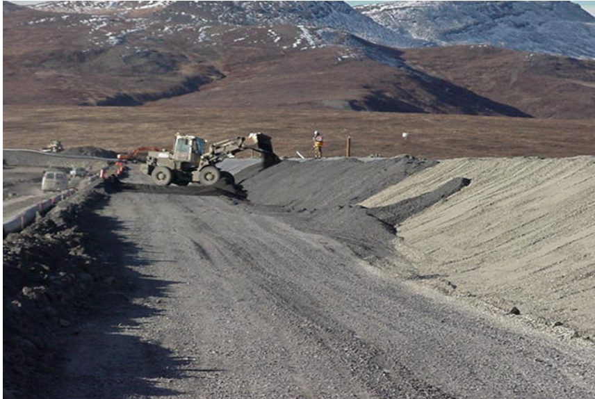
Placement and Grading of Liner Cover
