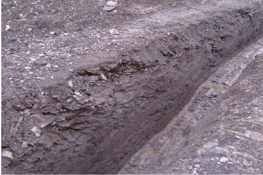
South Face & Bottom of New Cutoff Wall Excavation
