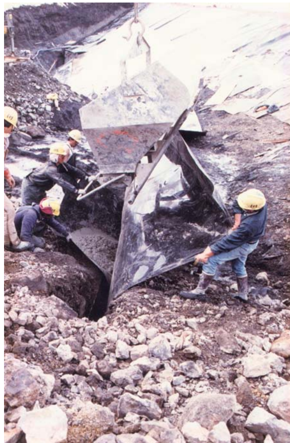
Cutoff Wall below Bottom of Cutoff Trench to Better Bedrock
