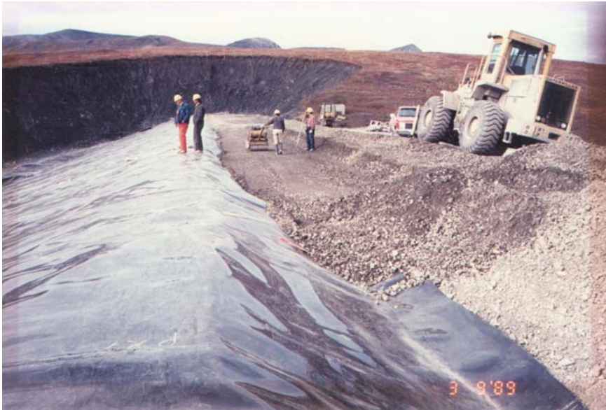
Anchor Trench Backfill at Top of Dam
