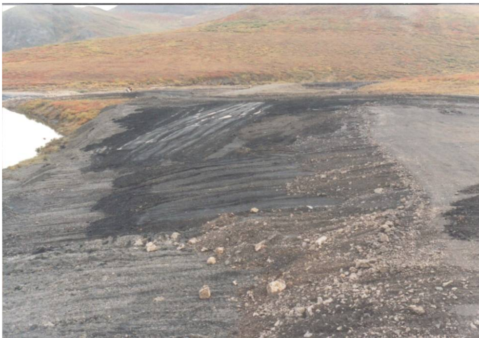
Left shoulder of Starter Dam Sta. 11+00 looking to the north. Edge of lift placed August 16 and 17, random rock from millsite.
