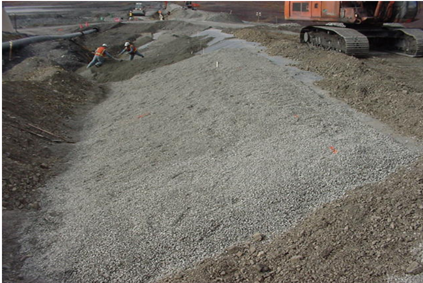
Cover Material over Geomembrane
