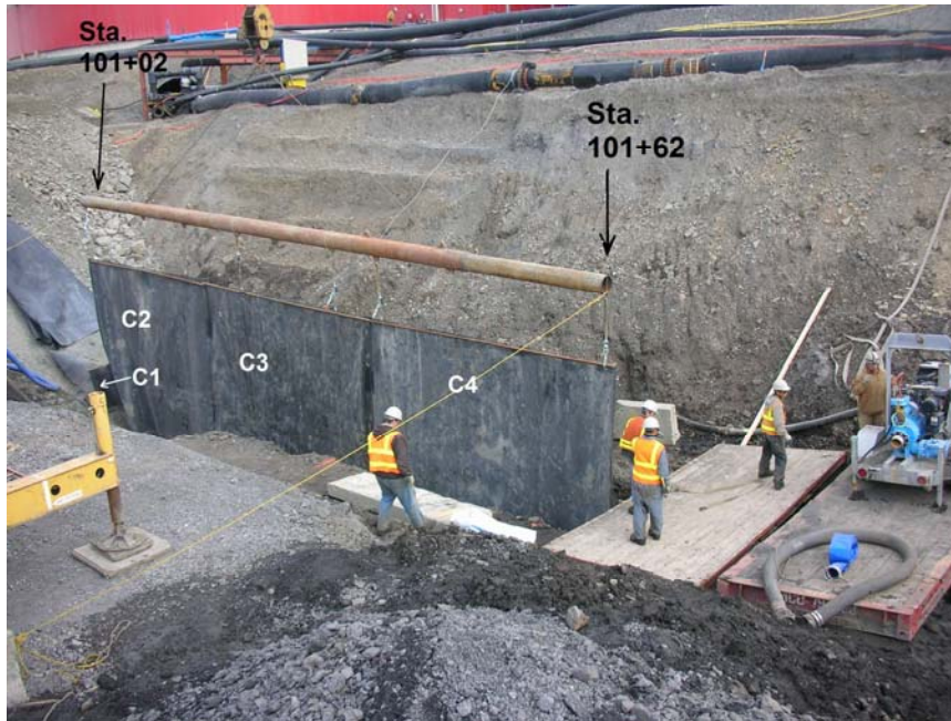
Curtain Wall First Four Panels
