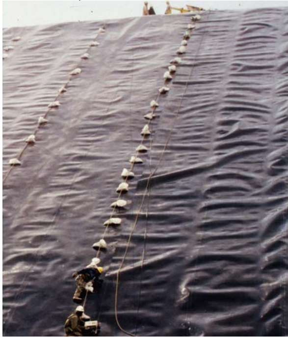
Geomembrane Panels and Seams Held Down
