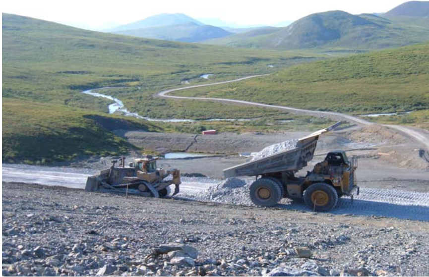
Widening Downstream Slope of Dam
