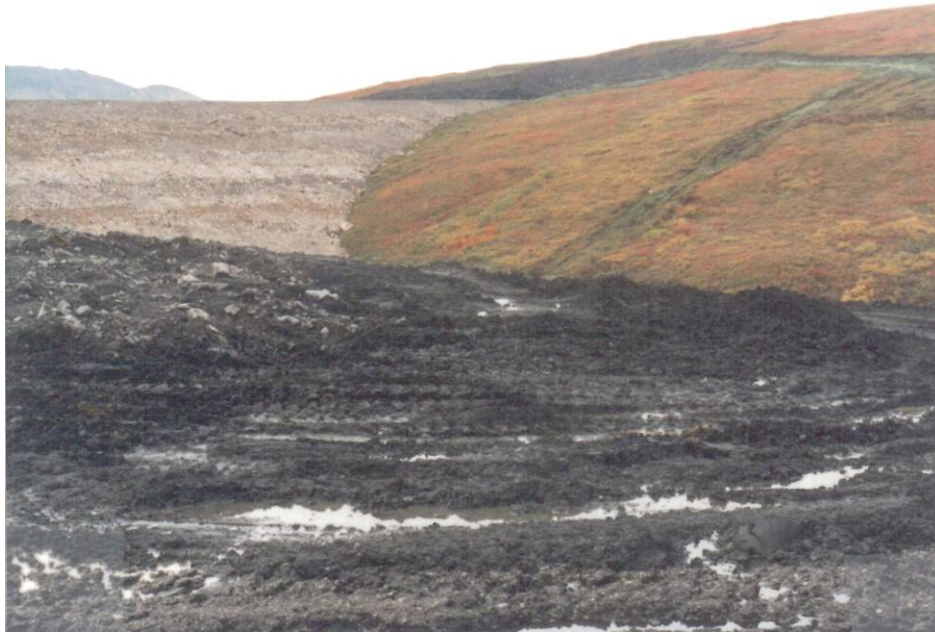
Taken from the seepage dam access road looking towards the starter dam. Area where D6 got stuck. Random rock fill placed over very soft and wet silty material.
