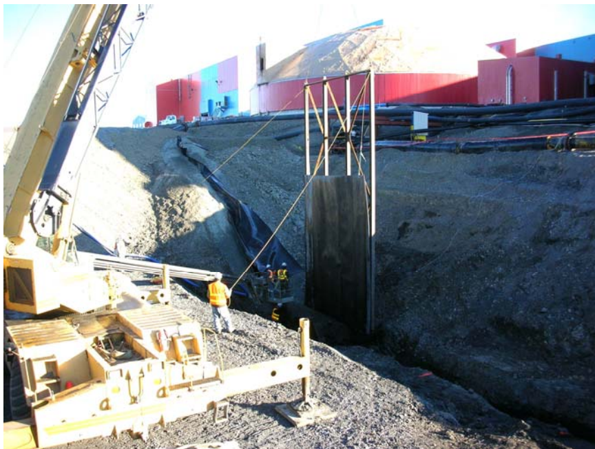
Curtain Wall Panel Insertion
