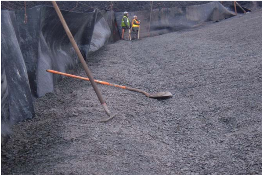
Liner Berm Fill at Toe of Cutoff Trench
