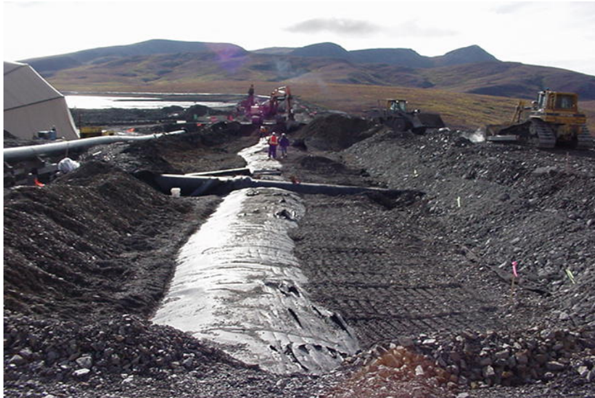
Stage VI Liner after Surface Scraped Off
