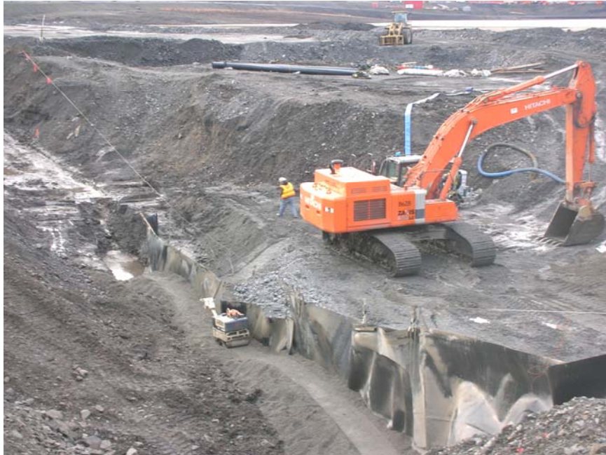
Curtain Wall Backfill and Continuation
