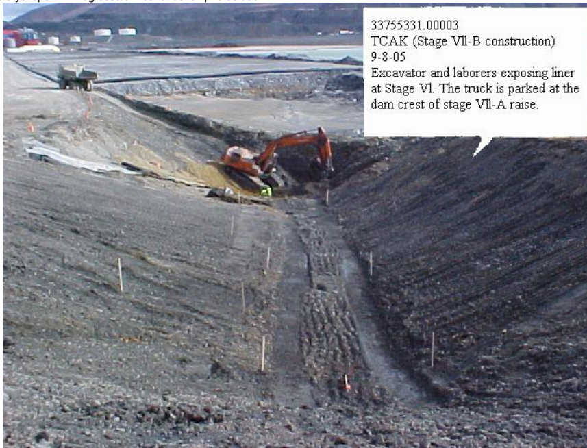
Exposing Stage VI Geomembrane for Cutoff Wall Extension
