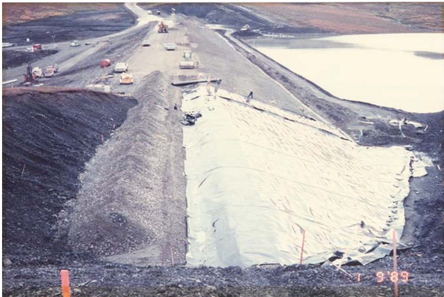
Liner and Anchor Trench
