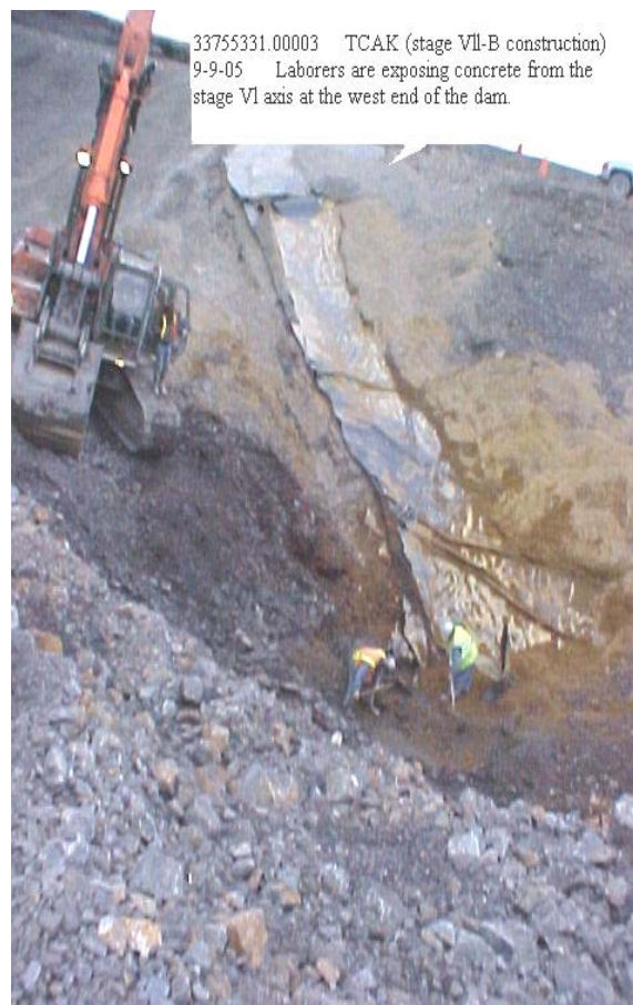
Exposing Stage IV Cutoff Wall and Stages IV, V, VI & VII-A Liner
