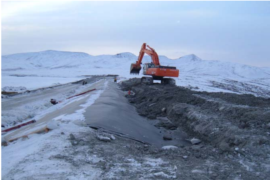
Backfilling Anchor Trench at Top of Dam
