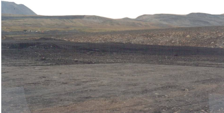
Fill material placed August 20, from millsite excavation (highly weathered/high moisture content).
