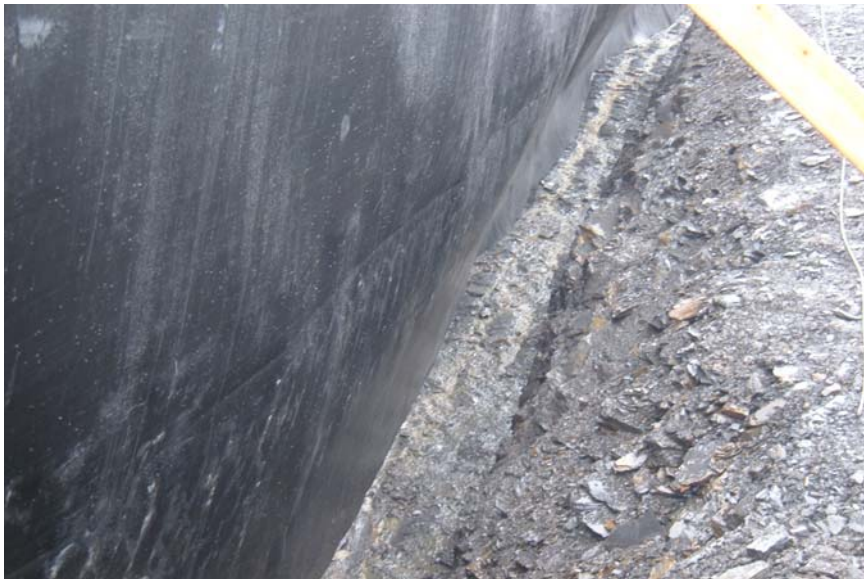
Excavation & Geomembrane for Cutoff Wall
