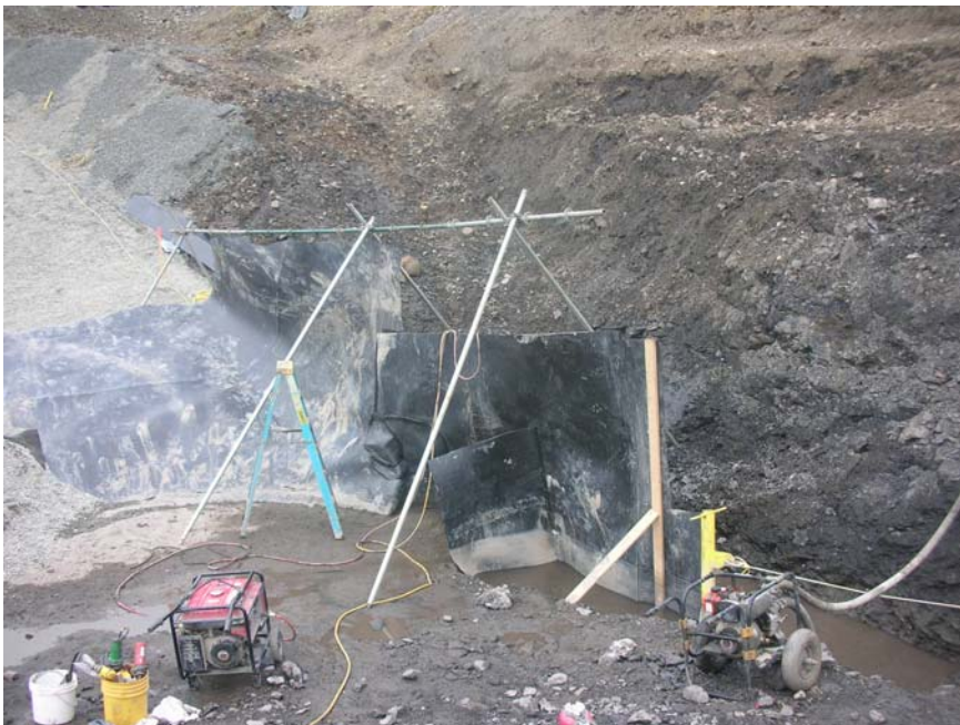
Liner System to Curtain Wall Transition
