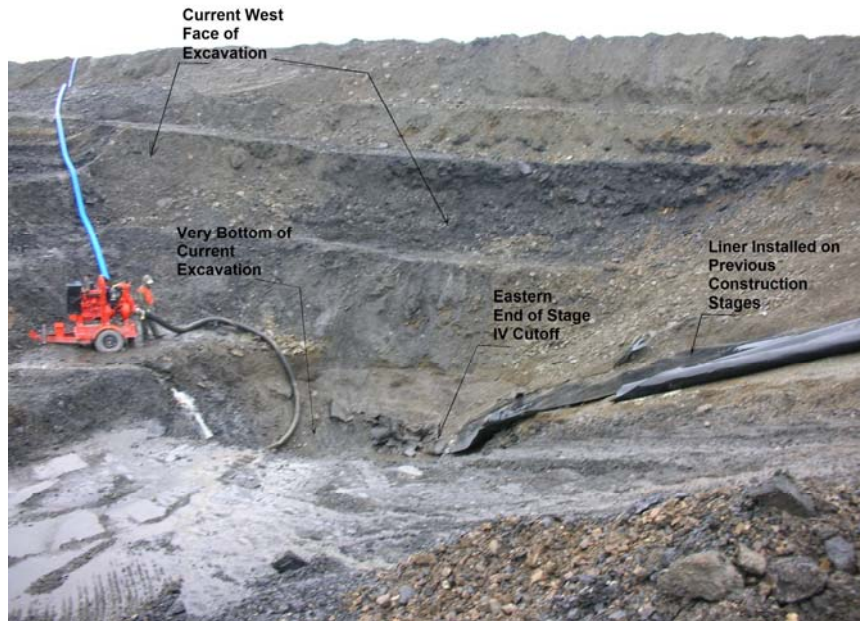
Cutoff Wall to Curtain Wall Concrete Tie-in
