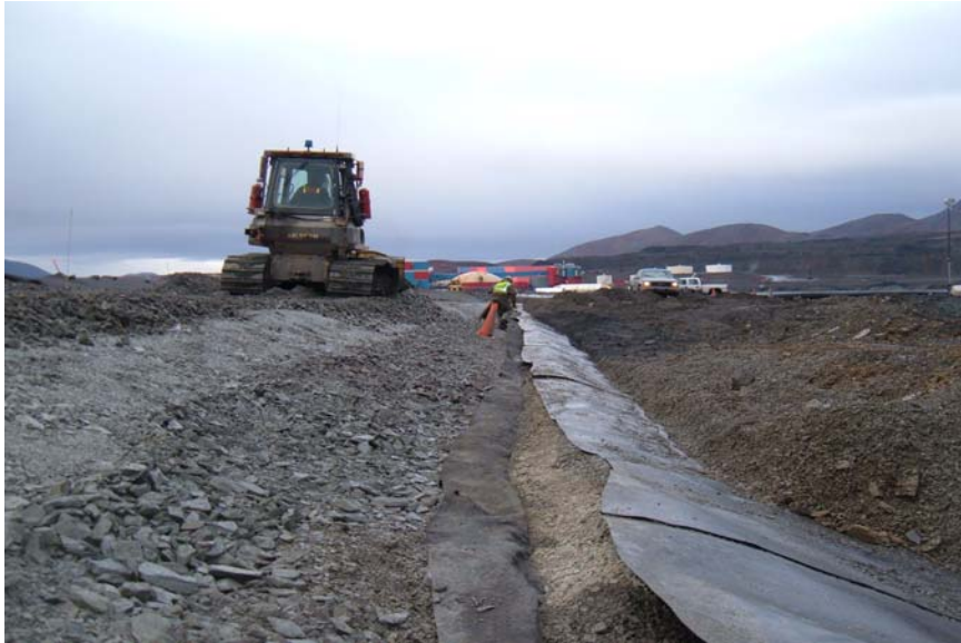
Exposed VII-A Geotextile, Bedding & Geomembrane
