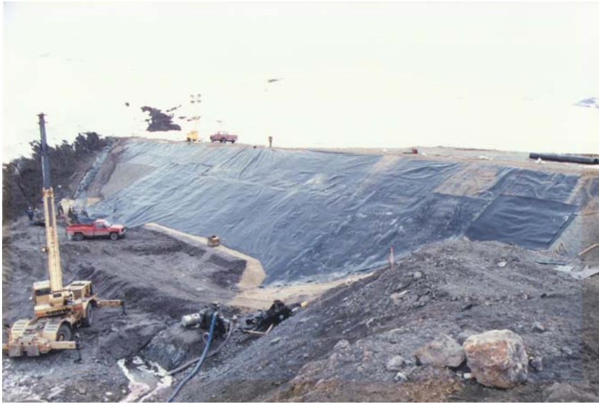
Upstream Face of Dam - Liner & Cutoff Trench
