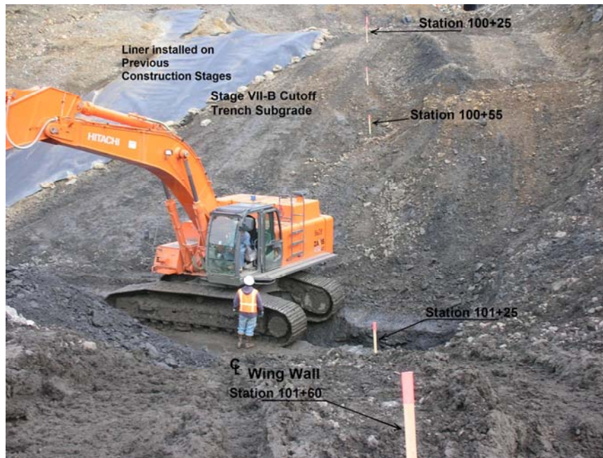
Start of Curtain Wall Excavation
