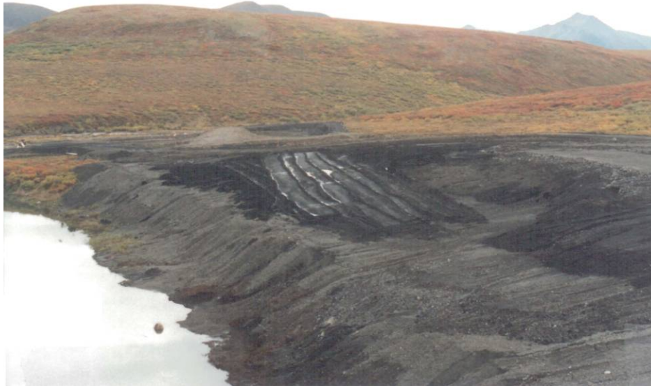
Left shoulder of Starter Dam Sta. 9+00 looking to the north. Polishing pond in top part of photo. Observe standing water on top of Stage 2 material.
