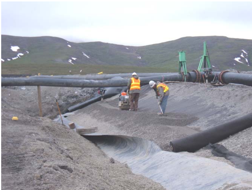
Bedding Around Relocated Pipelines
