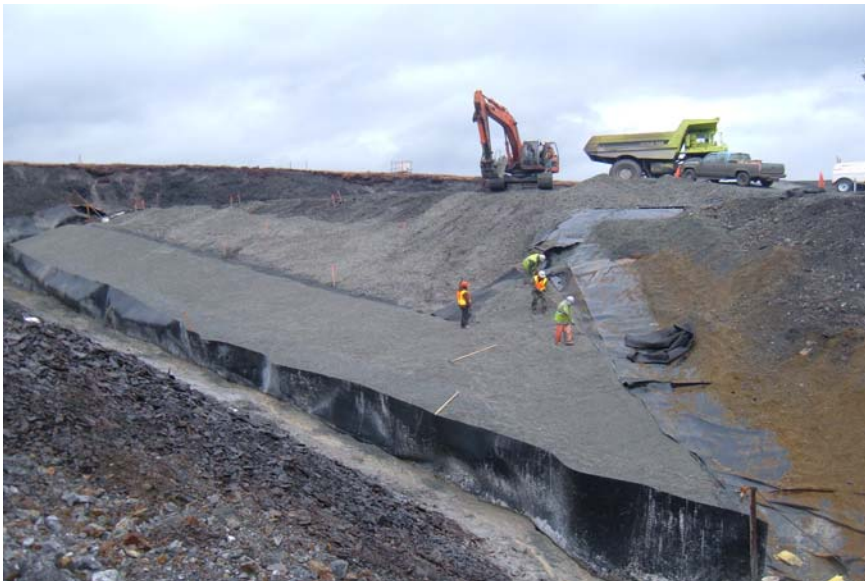
Fill to Cutoff Trench Subgrade
