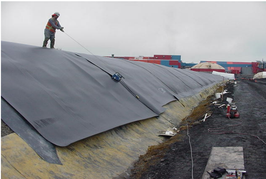
Vertical Seam between Geomembrane Panels
