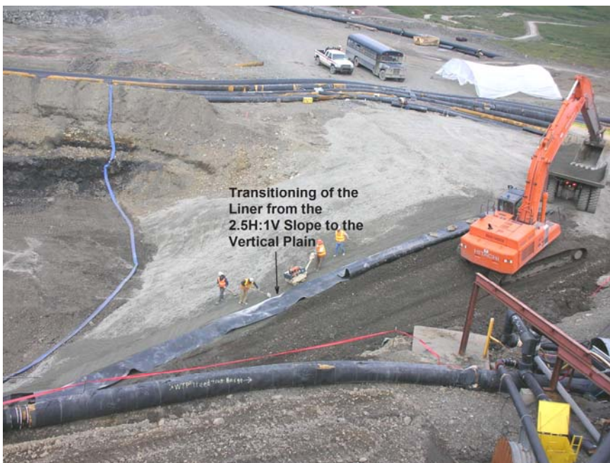
Liner Sloped to Vertical Transition
