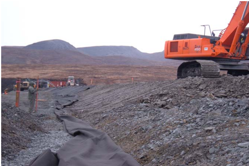
Placing Geotextile over Fill
