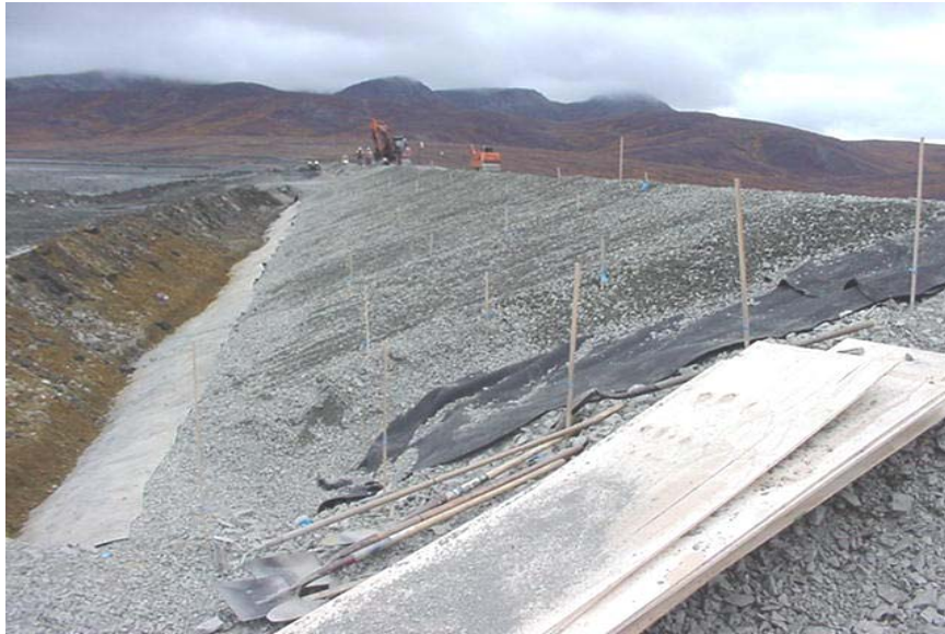
Bedding for Geomembrane Placement
