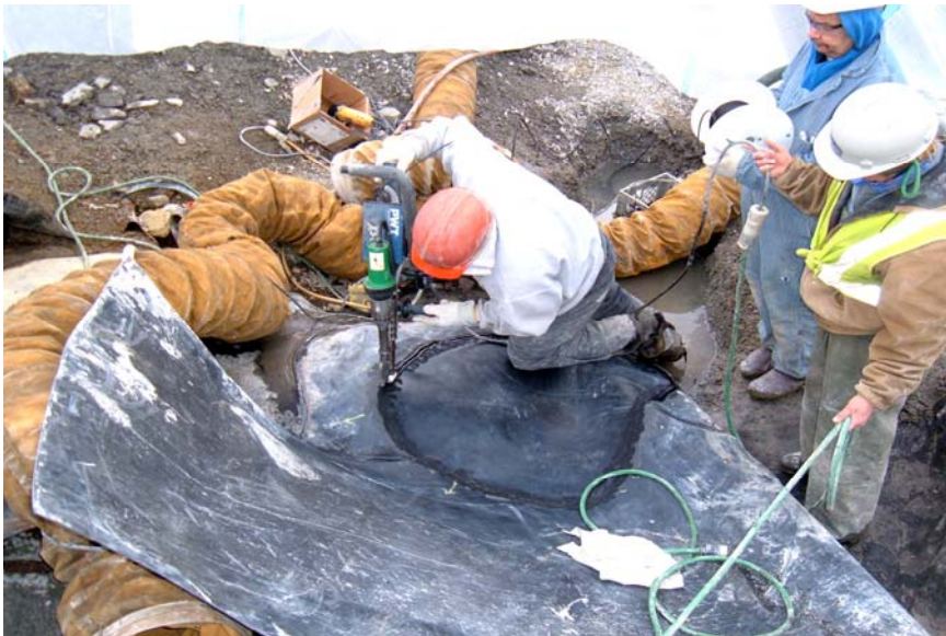
Welding in Stage VII-B Cutoff Trench
