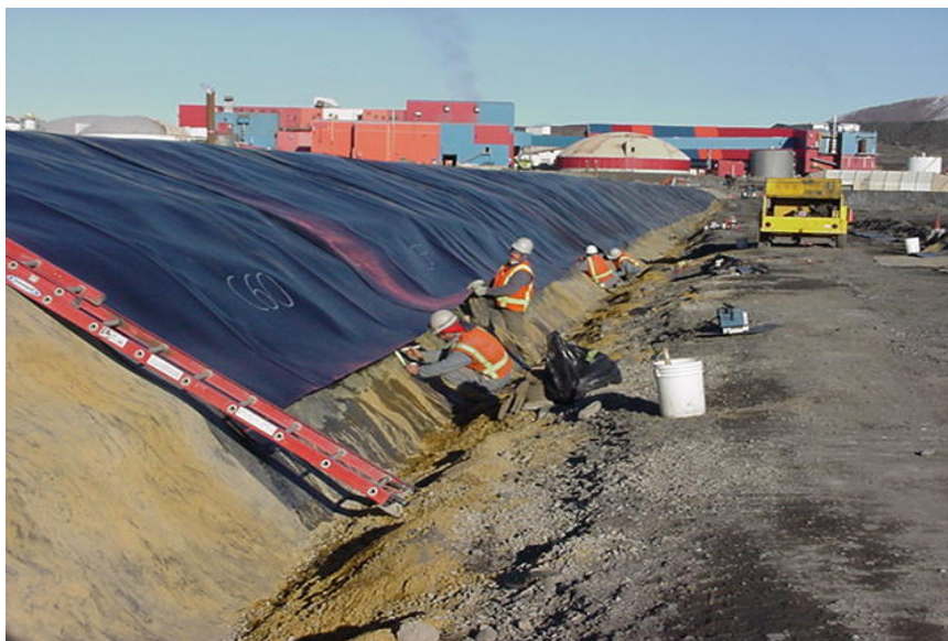
Welding New & Old Geomembranes
