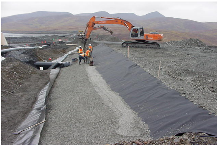
Bedding between Geomembrane & Geotextile
