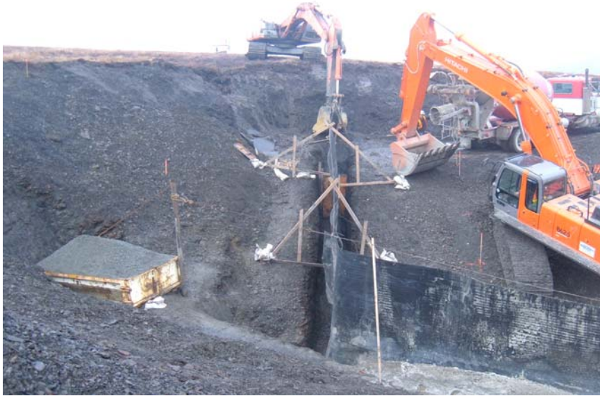
Cutoff Wall Extension at Left Abutment
