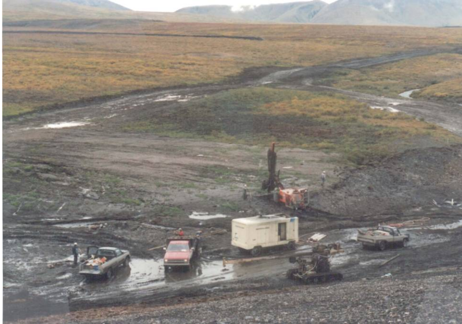
Right shoulder of starter dam. Crest, thermistor locations; T-11 to right of the black pickup in right corner, individual placing string; T-10 in the area of the Tamrock; T-9 left corner of photo with white PVC above ground.
