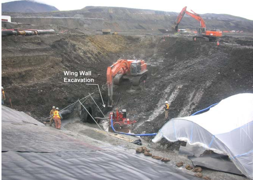
Curtain Wall Start of Excavation
