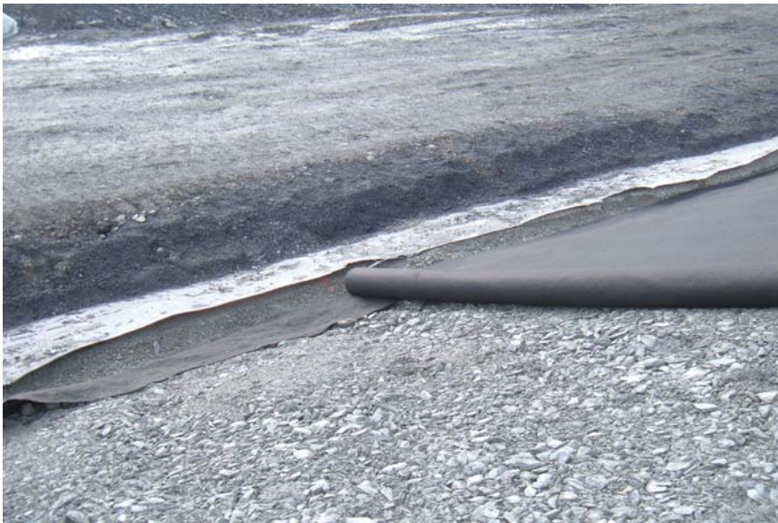
Type II Geotextile over Type 3 Fill
