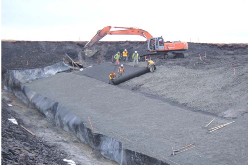
Geotextile on Cutoff Trench Subgrade
