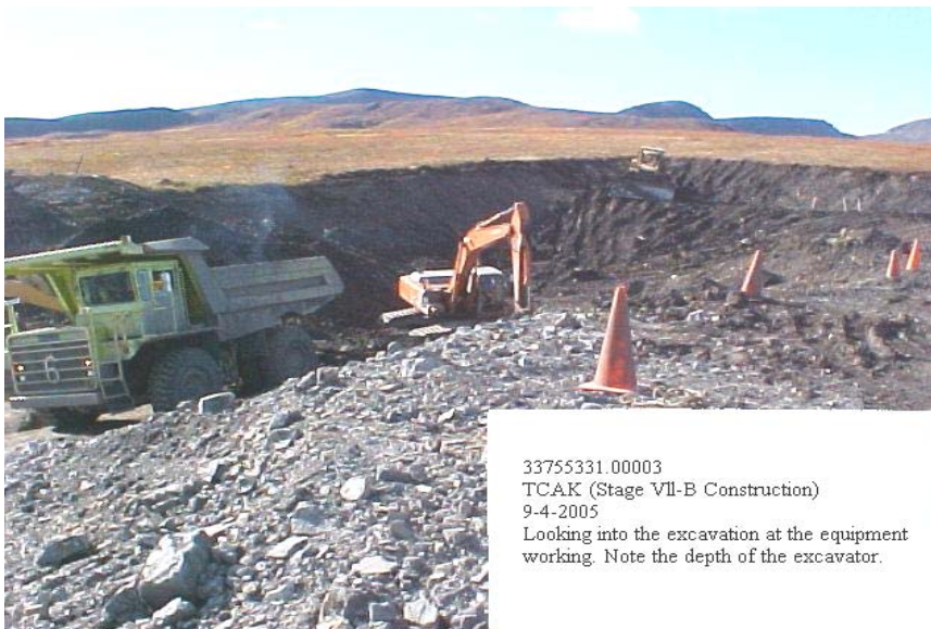
Excavating Left Abutment to Cutoff Trench
