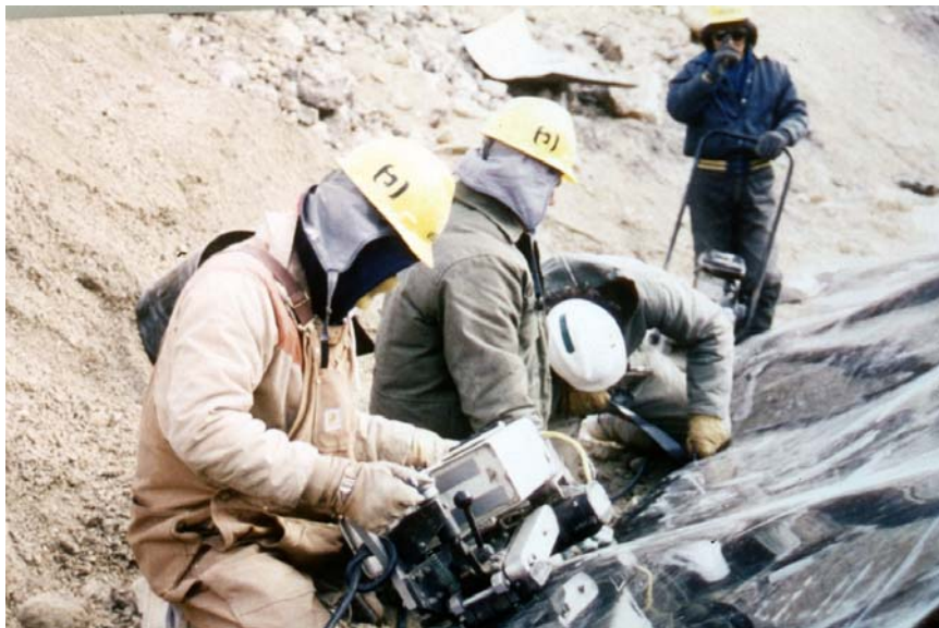
Geomembrane Panel Seam Welding
