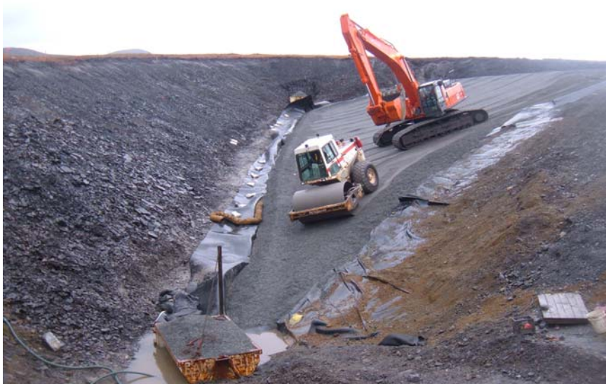
Fill in Cutoff Trench for Geomembrane Installation
