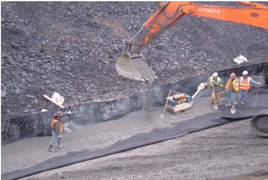
Fill on Geotextile at Toe of Cutoff Trench Subgrade
