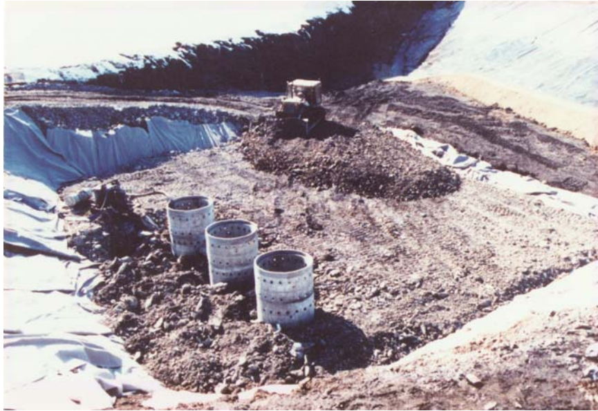
Pumpback System in Seepage Collection Pond
