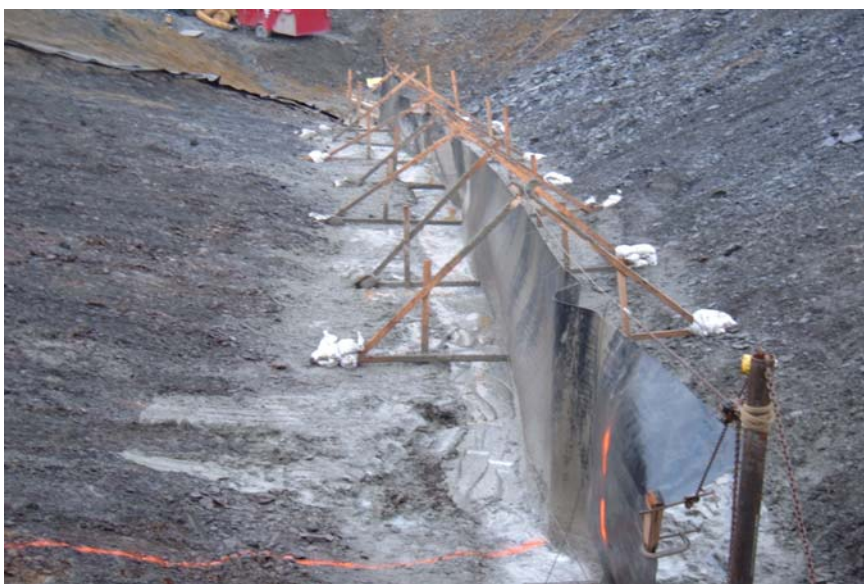
Grout Poured to Top of Cutoff Wall Excavation
