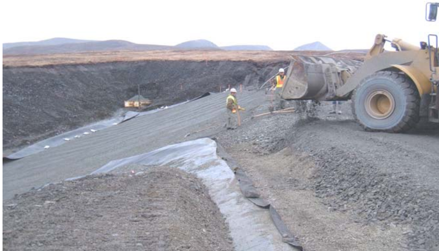
Placing Fill for Geotextile Installation
