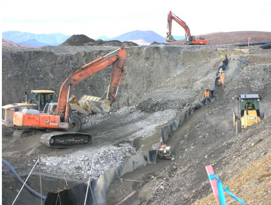
Curtain Wall Backfill Up Abutment
