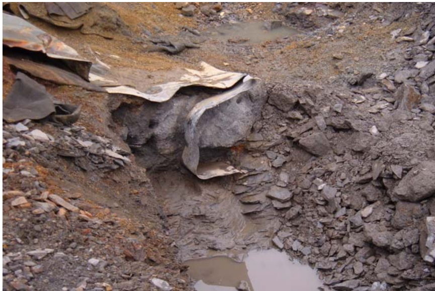
Exposed End of Stage IV Cutoff Wall
