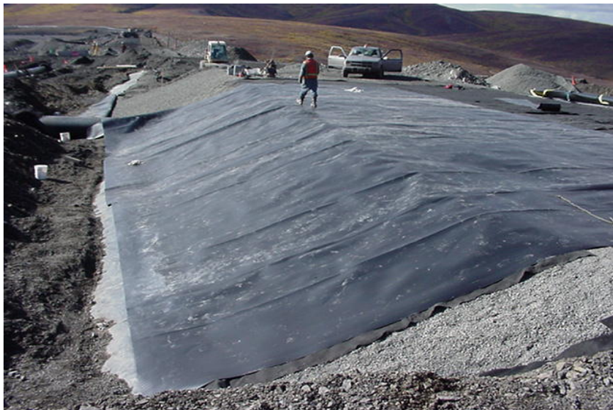
Geomembrane on top of Bedding
