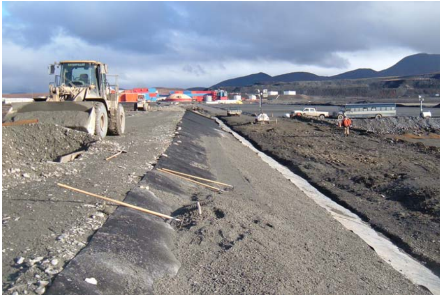
Extending Geotextile & Liner Bedding up to El. 960
