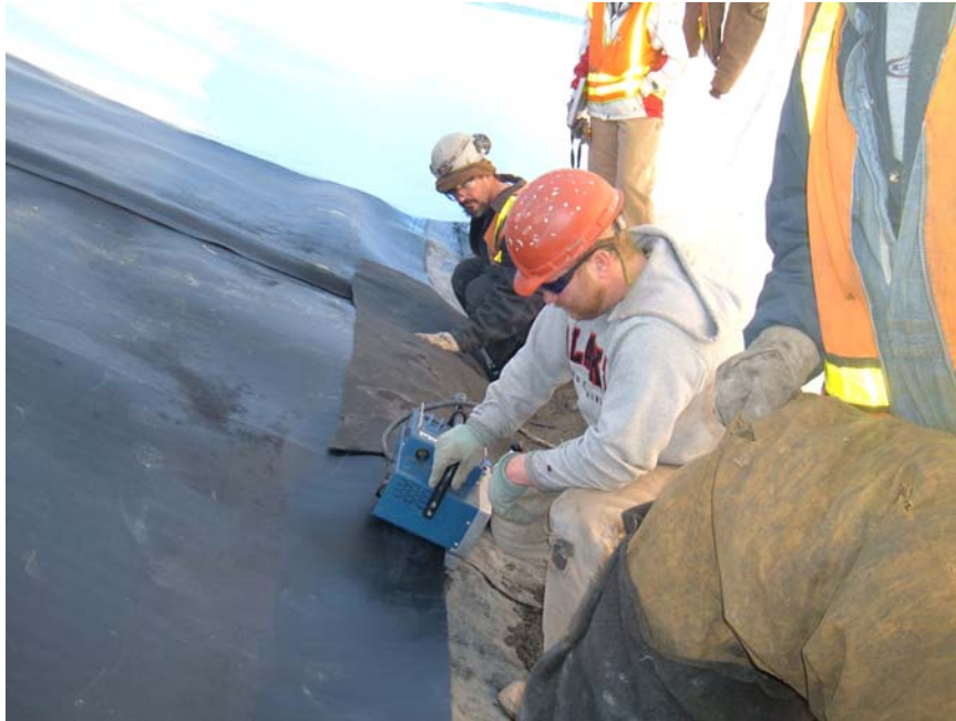
Seam Welding between Stage VII-B & A Geomembrane
