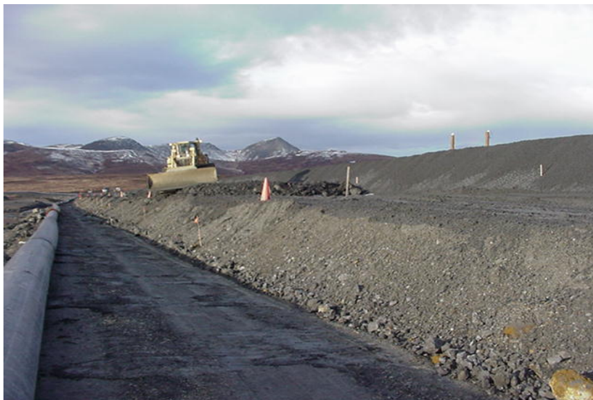
Placement of Buttress to Protect Liner
