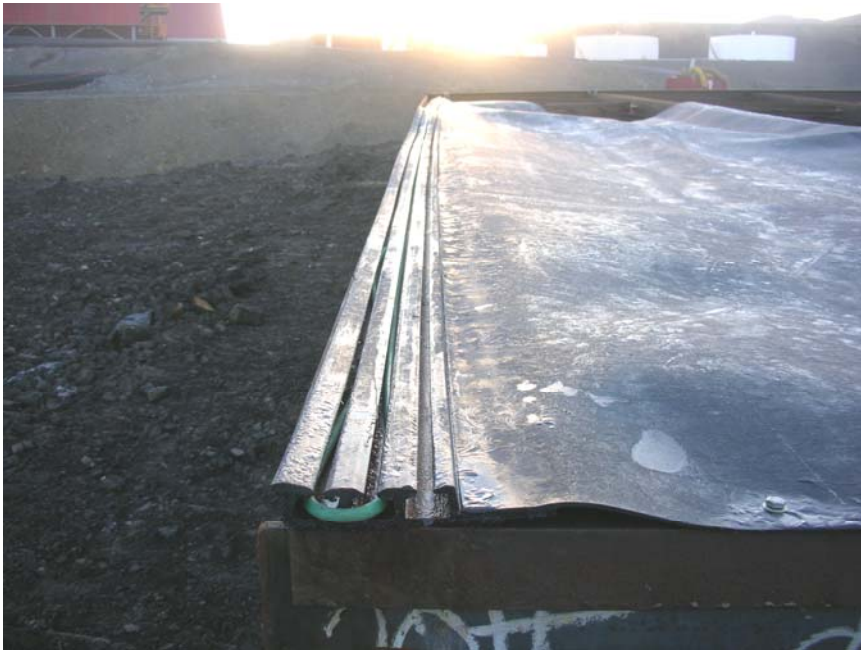
Curtain Wall Panel Interlock
