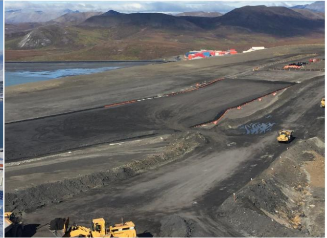
Photo 2 – Looking northwest at the top of the MWD.
