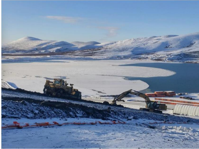
Photo 1 – Looking west off MWD. Placing cover rock over the geocomposite.
