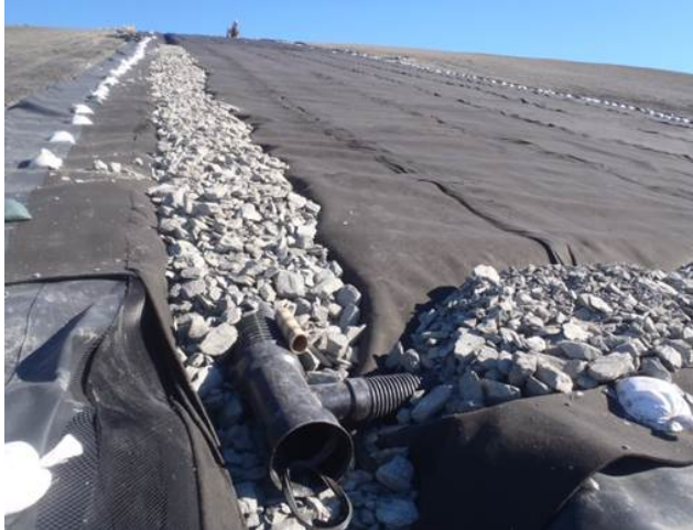
Photo 2 - Two acre test, MWD toe, west face looking east, final placement of drainage mat over LLDPE, prior to placing 2 feet of cover rock on top.
