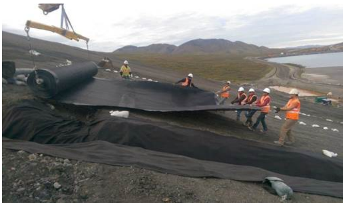
Photo 1 - Two acre test, Looking south, near south end of MWD. Placing double textured LLDPE on MWD surface.
