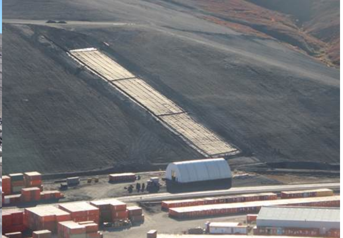
Photo 3 - Two acre test, aerial of cover construction
