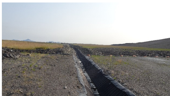
Water collection ditch on Main Waste Dump
