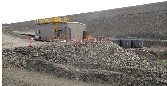
New Seepage Collection system below downstream face of the Main Dam
