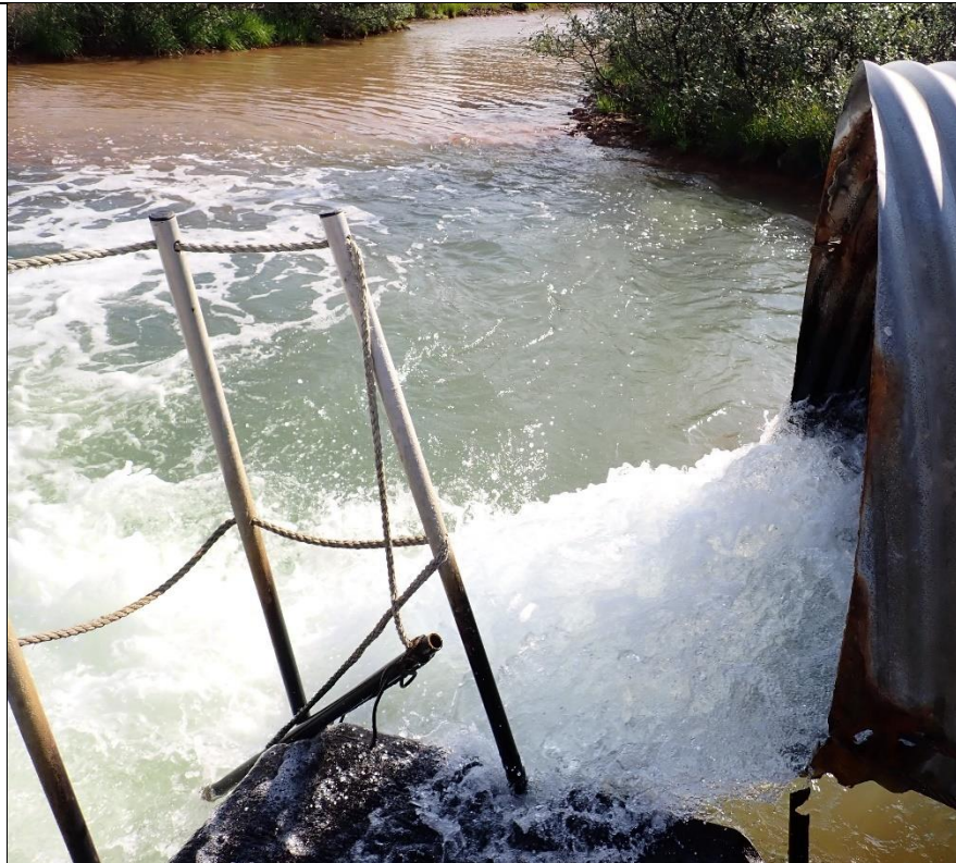
Photo 5: Treated water discharge flowing into Red Dog Creek. Notice the change in water clarity between the mineralized background water flowing into this mixing zone.
