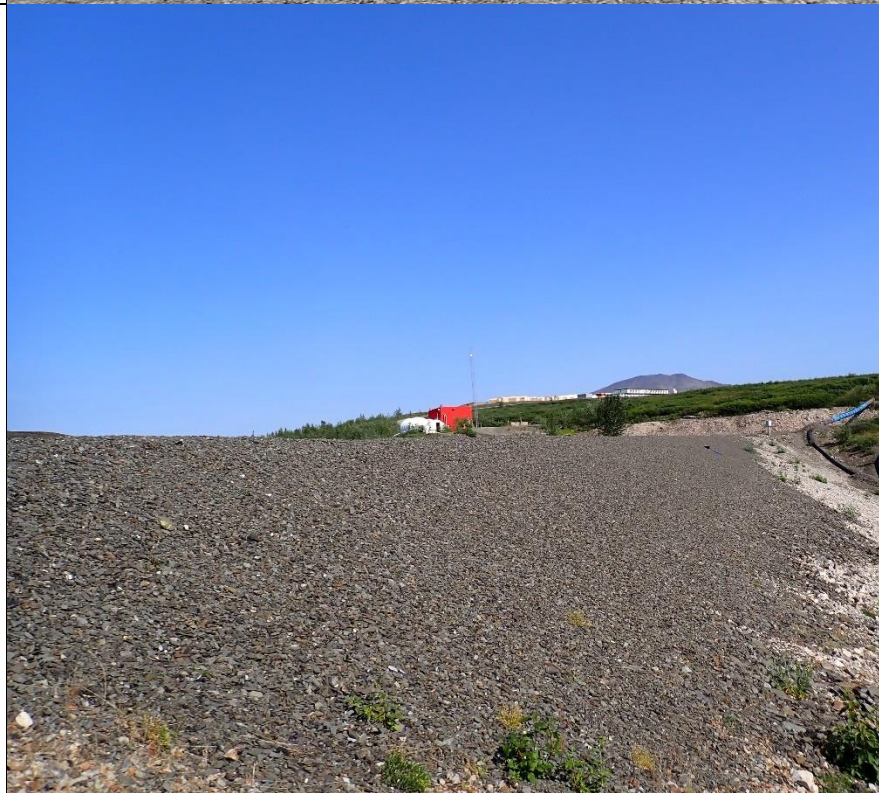
Photo 22: Bons Reservoir dam (center) and freshwater pump station for mine (above).
