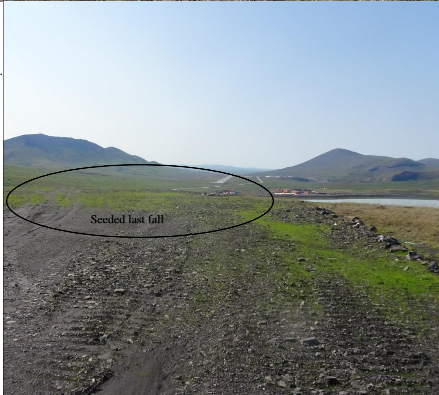
Photo 12: View looking south at the main WRD that was seeded in the fall of 2023. Just to the right is the plot that was seeded in 2017. Notice the rate of growth and dispersion.
