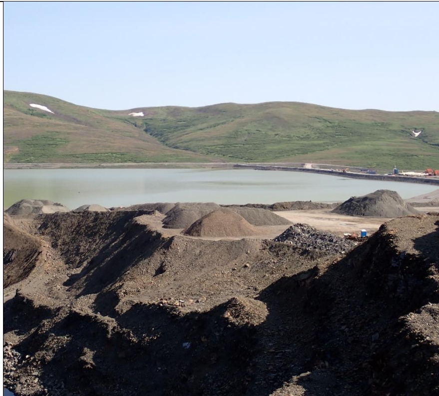
Photo 23: DD2 material site stockpiles.
