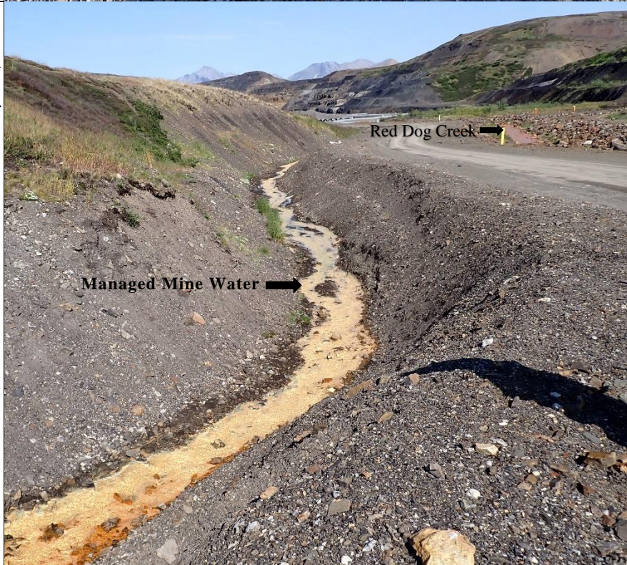
Photo 16: Water captured from the drainage off the back side of South Qanaiyaq Pit. Ditch (Center) is part of the mine water management. Upper right of photo is Red Dog Creek that is separate from the managed mine water.
