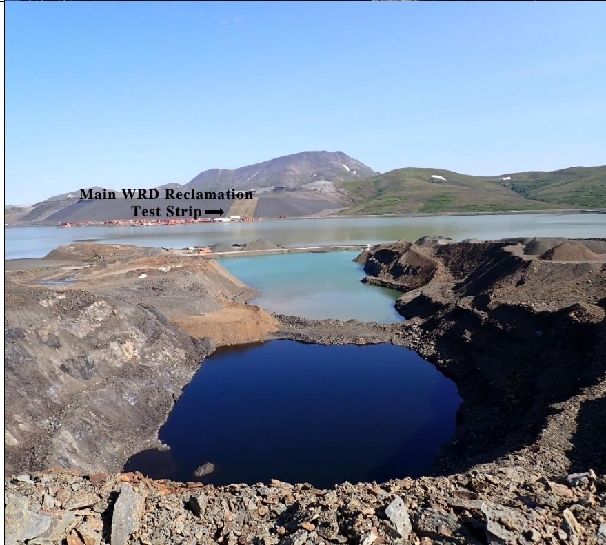
Photo 24: Pits of DD2 have infilled with water which lie adjacent to the southwest side of the TSF. The main WRD (background) can be seen for perspective. Most of the surface area of the WRD has been graded with growth medium.
