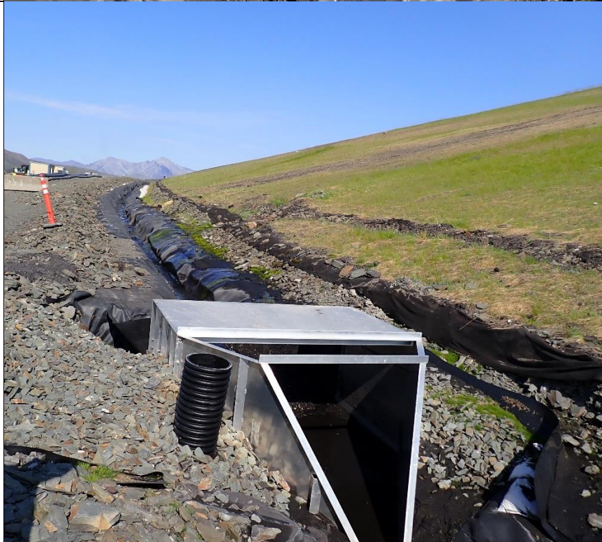
Photo 20: View of the ditch looking north, 180° degrees from Photo 19. No topsoil debris accumulation in ditch from erosion. Right side of photo is the 17-acre reclamation seeded in 2017.
