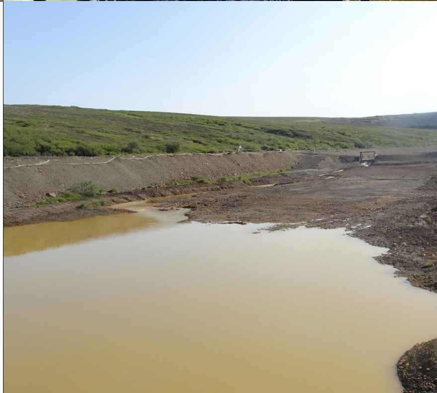
Photo 6: Main mine sump with water actively flowing in. This water is pumped from collection points within the mine to the TSF.
