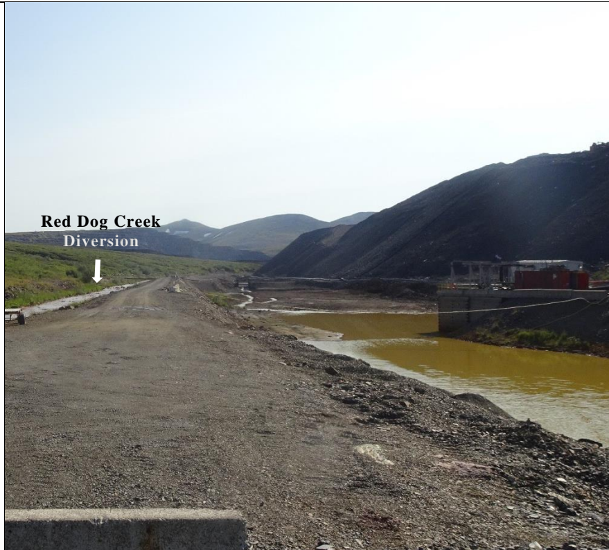
Photo 7: View of the mine sump impoundment. The water volume is above what has been observed during previous inspections. Red Dog Creek diversion runs adjacent to the mine sump returning to its original channel just downstream of the sump impoundment.
