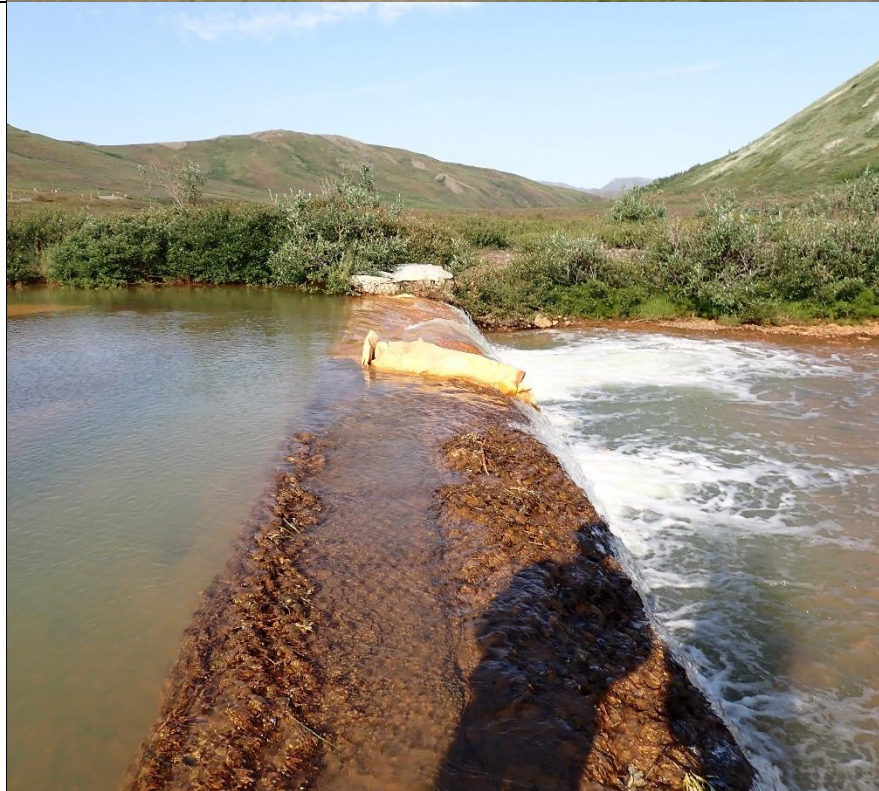
Photo 4: Fish weir located downstream from the mill discharge point on Red Dog Creek. Notice some of the sheeted material has dislodged. On previous inspections, the entire weir was covered.
