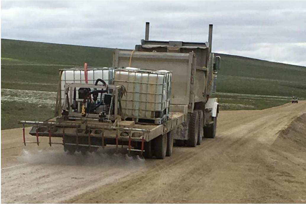
Figure 1 Photo of the ESprayer System. Totes containing EK-2800 loaded on the trailer.
