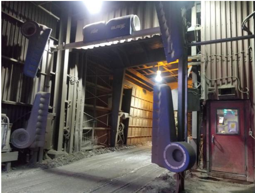
Photo 1. Six blowers installed inside the Truck Unloading Building.
