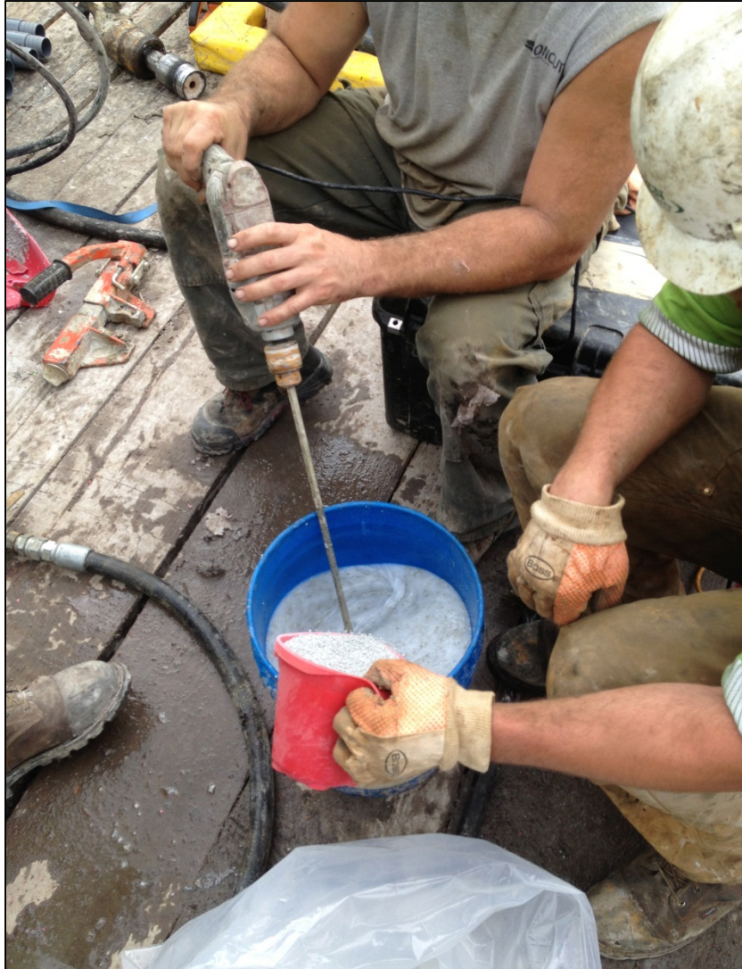
Mixing EZMud polymer grout for seal in cement basket and around benseal sleeves
