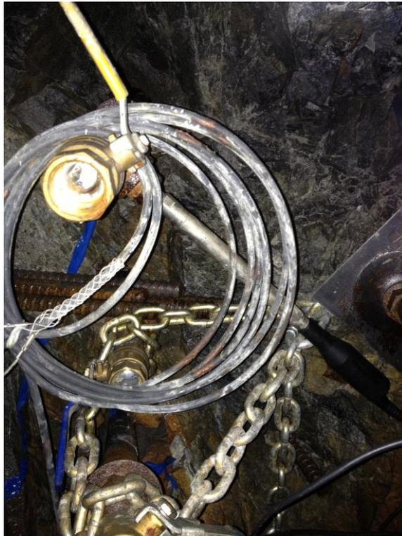
Picture 2: Final set up of margot plug
