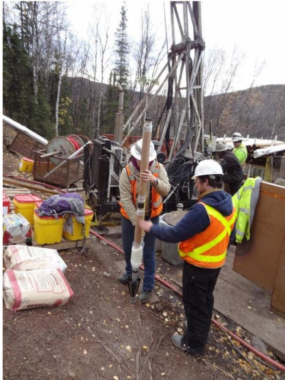
Picture 7: Assembling Cement basket, and Benseal Sleeves
