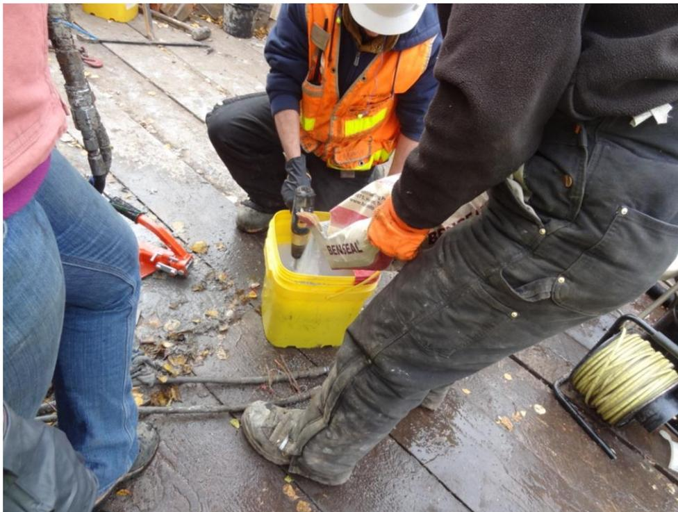
Picture 13: Mixing benseal slurry. Will cure the benseal sleeves.
