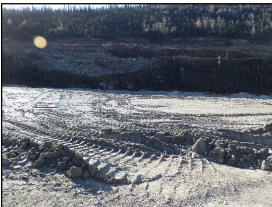
Photo 13: Dry stack tails section regraded.
