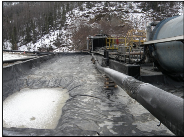
Photo 9: East side of paste backfill secondary containment
