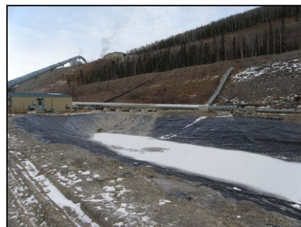
Photos 13 & 14: Storm Water Sedimentation Pond
