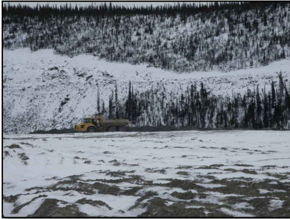
Photo 15: Truck unloading tailings on DSTF
