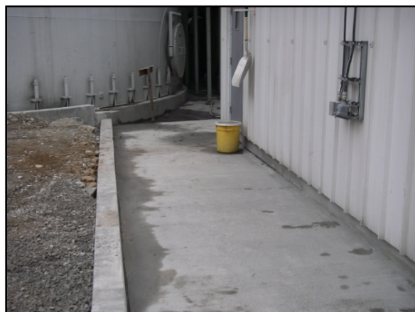
Photo 26: New cement pad and curb outside paste building
