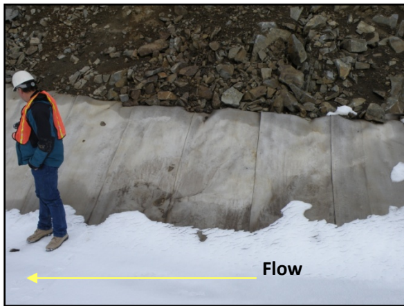
Photo 21: Section of new liner segments
