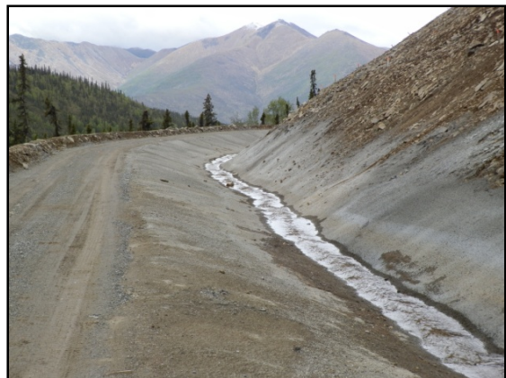
Photo 2: Water flowing down the shotcrete-lined North Diversion Ditch.
