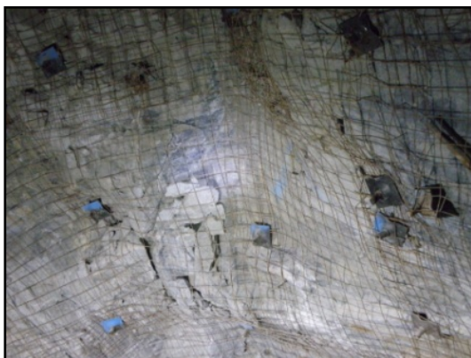
Photo 5: Completed section of roof rock bolting.
