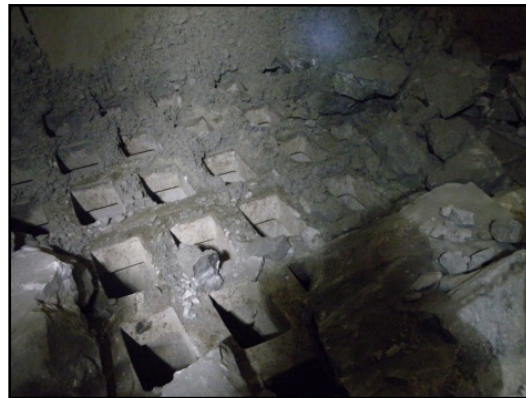
Photo 10: View of the grizzly for the ore pass.
