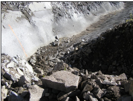
Photo 17: A view of the old north drainage ditch.
