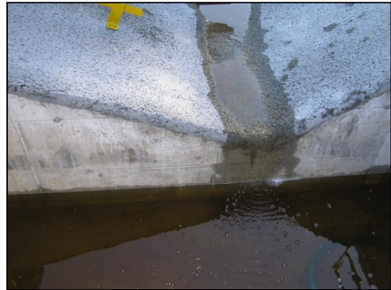
Photo 24: Drainage channel constructed for flow into the south flume sump.
