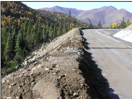
Photo 29: Berms are maintained along the mine roads.
