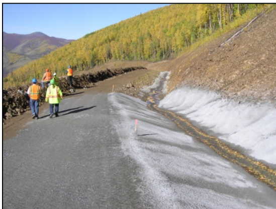
Photo 11: North side connection between the old and the new diversion ditches.
