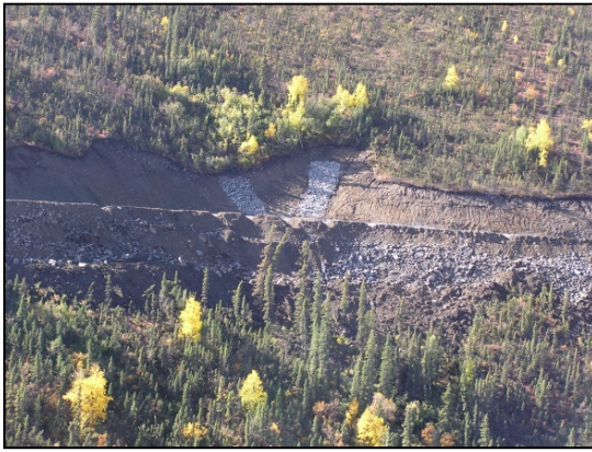
Photo 15: A view of drainage channels for surface streams on the south side.
