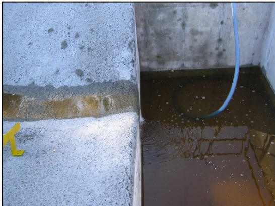
Photo 23: A view looking into the south flume sump.
