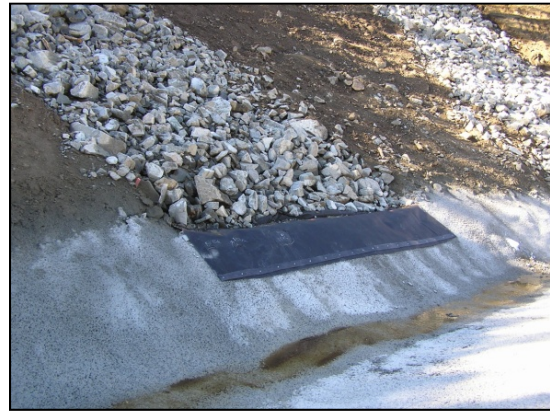
Photo 16: The stream intercept on the south side drainage ditch.
