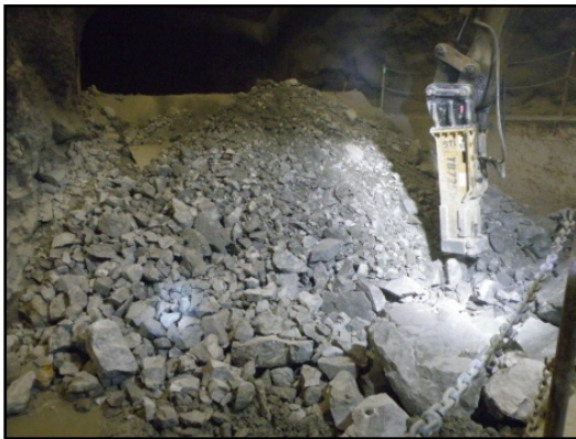
Photo 9: Rock breaker in action.
