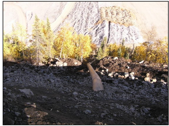
Photo 20: A view of the drop pipe to connect the new south ditch to the old north ditch.
