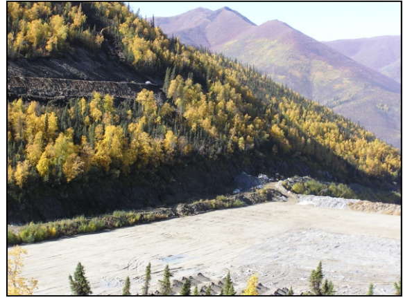
Photo 26: An overview of the area where the south diversion ditch systems are tied together.
