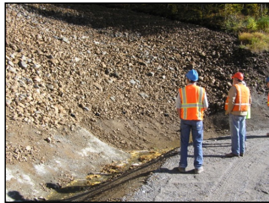
Photo 12: One stream channel intercept with the north diversion ditch system.
