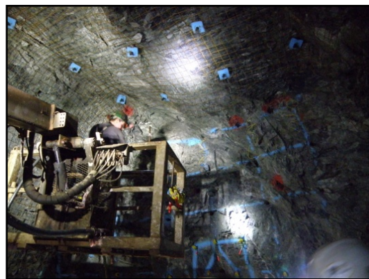
Photo 6: Blaster loading holes for the next shot.
