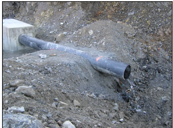
Photo 22: A view of the exit from the south diversion ditch pipe.
