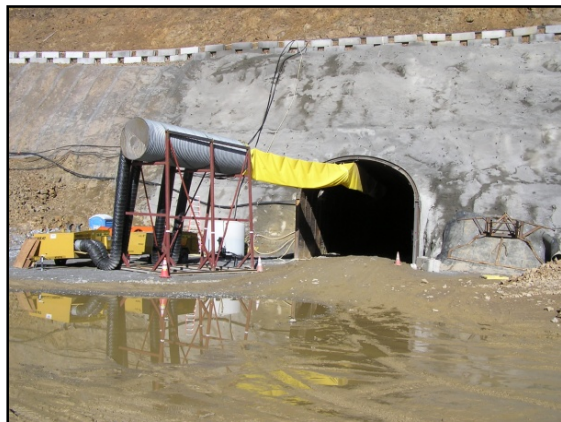
Photo 27: Ventilation installation for the 2150 portal.
