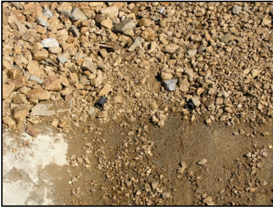
Photo 13: Stream channel #1 intercept with the north drainage ditch.
