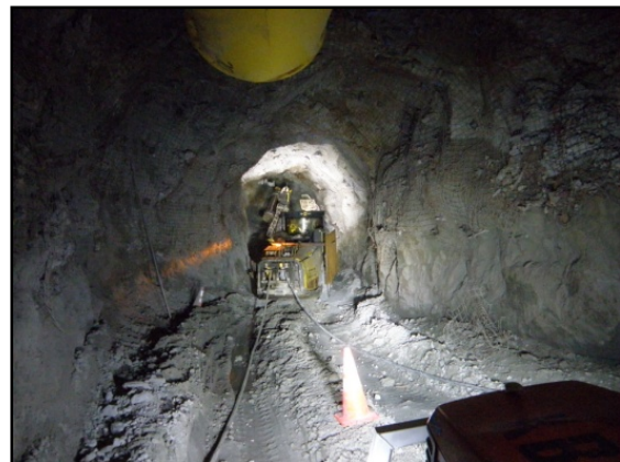
Photo 4: Rock bolting and underground support installation.
