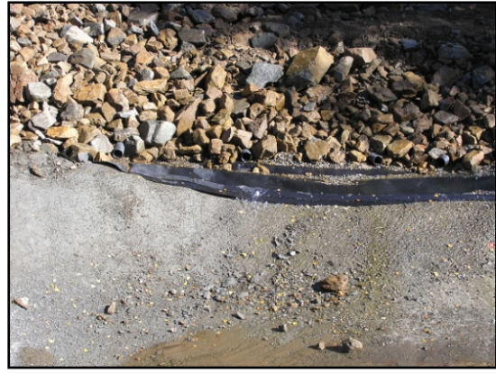
Photo 14: Stream channel #2 tie intercept with the north drainage ditch.
