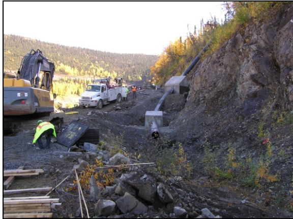
Photo 25: A view of the terrain and the south diversion ditch pipe system.
