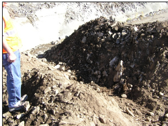
Photo 18: A view of the old north drainage ditch.
