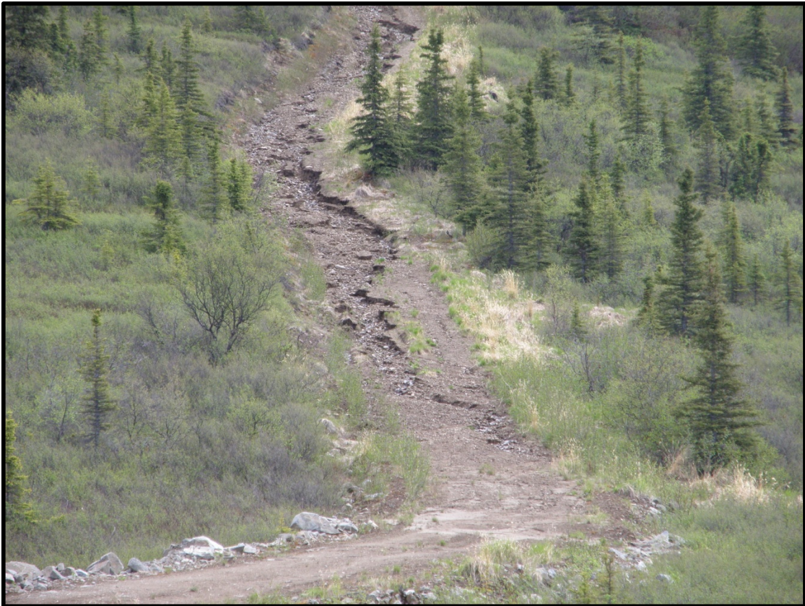
Photo 2 – Erosion of Communication Tower Access Road
