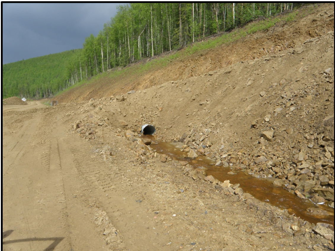
Photo 5 – Culvert and Access Crossing Old Diversion Ditch to New Diversion Ditch
