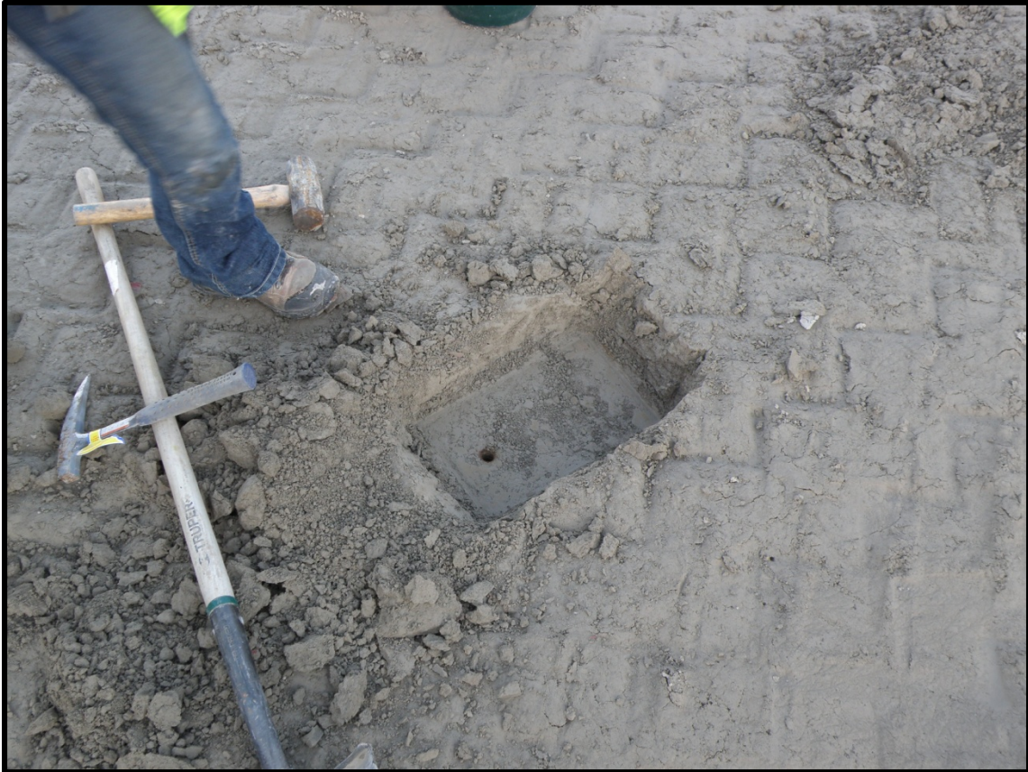
Surface and Probe Hole Prepared for Nuclear Gauge
