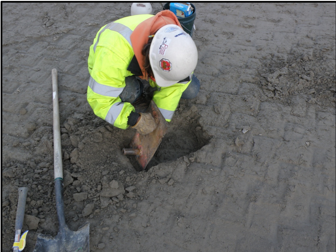
Preparing Surface for Nuclear Gauge
