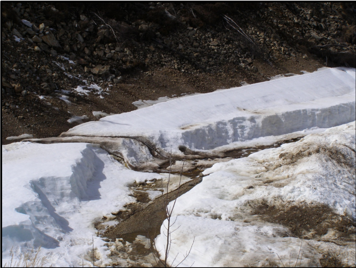
Photo 9 – Overflow from Upper Liese Creek into West Diversion Ditch
