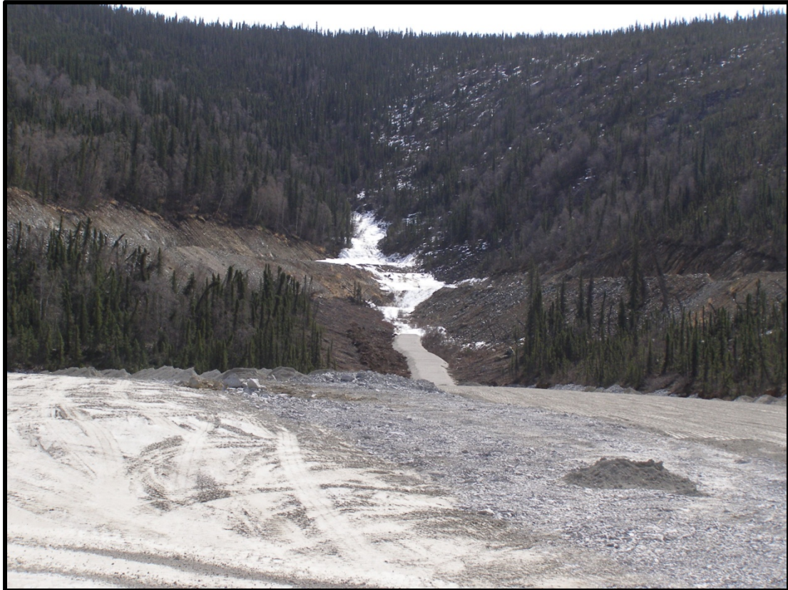
Photo 6 – Drystack - Compacted Tailings with Mineralized Rock in the Center
