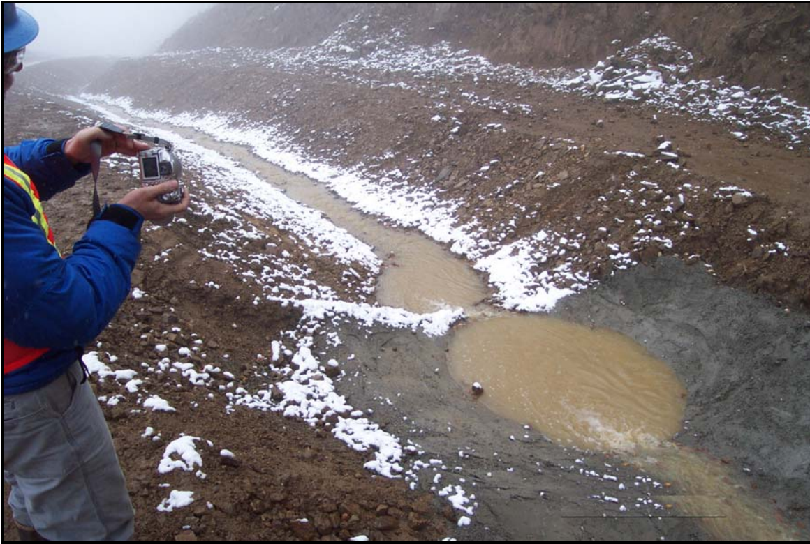
Photo 2 – Flow in diversion ditch on North Side of Liese Creek, disappears within 50 yards below shotcrete.
