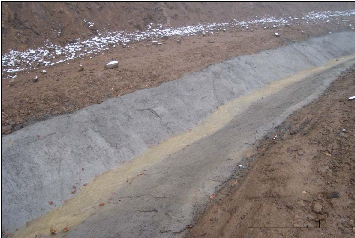
Photo 1 – Shotcrete lining in diversion ditch on North Side of Liese Creek.
