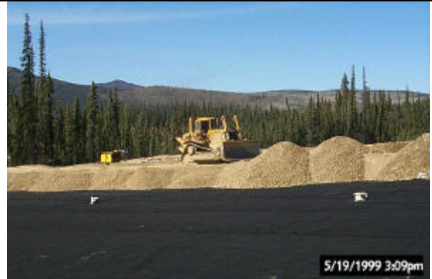
Figure 2. D-7 dozer spreading over-liner.
