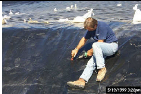
Figure 3. Lystering liner seam in ditch.
