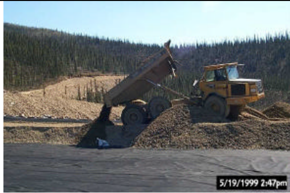
Figure 1. End dumping two-inch minus over-liner.
