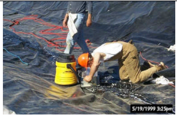
Figure 4. Vacuum testing of welded liner seam in ditch.
