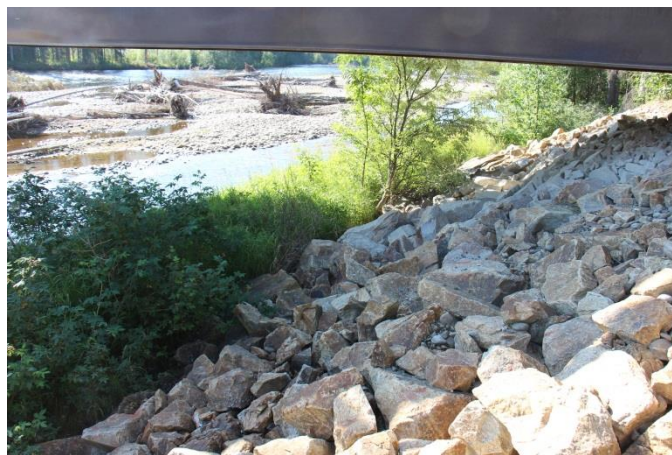
Photo 15. Goodpaster River Bridge Scour Protection, West Bank
