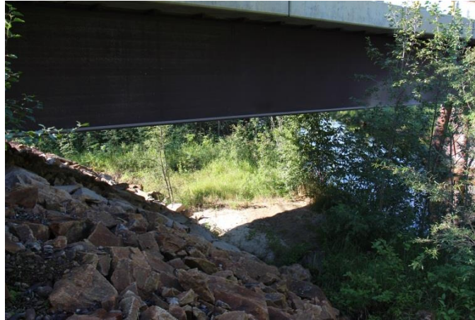
Photo 16. Goodpaster River Bridge Scour Protection, East Bank
