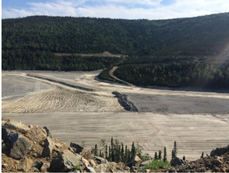
Photo 3. DSTF tailings compaction surrounding the mineralized rock disposal in the center of the facility. Non-mineralized rock disposal along margins of the facility.
