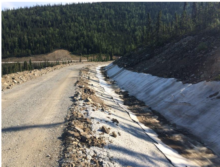
Photo 2. Diversion ditches carrying offsite flows around mine facilities, discharging to Liese Creek. Ditches are free from sediment or blockages, and Pogo is addressing erosion of slopes upgradient from the ditches.
