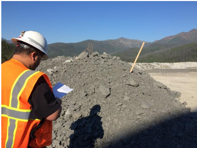
Photo 10. Waste rock outside of portal labeled with the survey lath and waiting for laboratory results for flagging before ultimate disposal.
