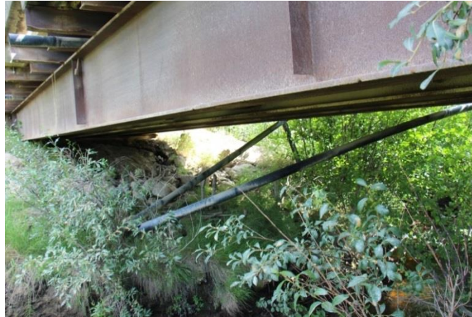
Photo 28. West Keystone Creek Bridge, East Bank Scour Protection
