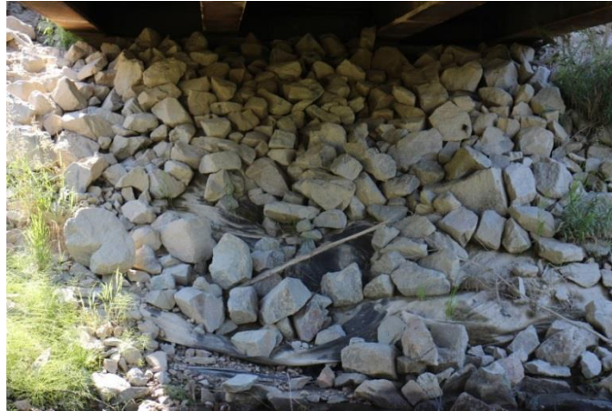
Photo 19. Shaw Creek Bridge, Degraded Scour Protection
