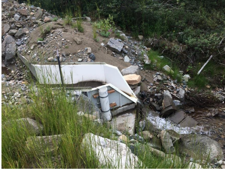
Photo 5. Flumes were intact and maintained free of debris or sediment.
