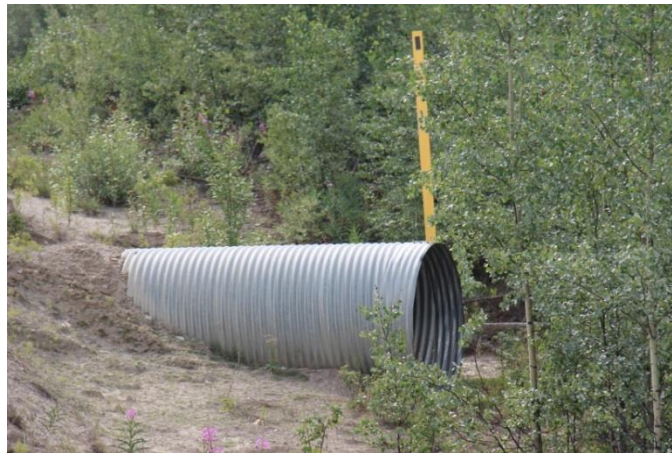
Photo 29. Typical Drainage Culvert
