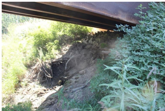
Photo 21. Gilles Creek Bridge, Abutment Scour, West Bank
