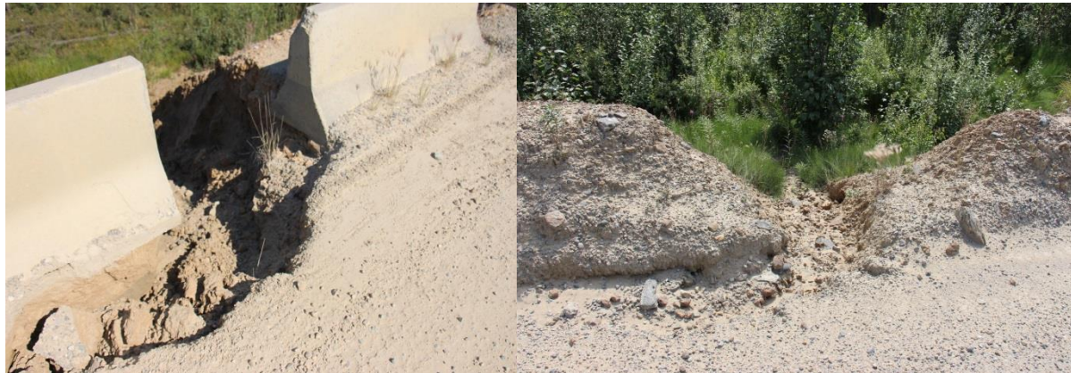
Photo 36. Erosion Caused by Roadside Barriers
