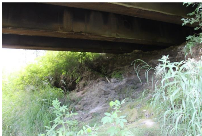
Photo 24. Caribou Creek Bridge, West Bank Abutment, No Scour Protection
