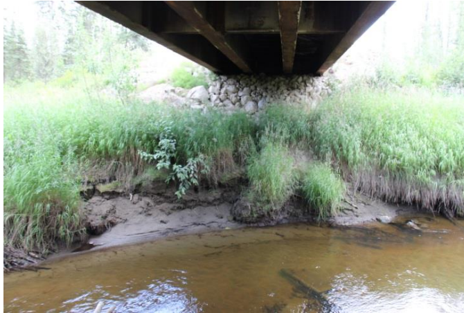
Photo 25. Caribou Creek Bridge, East Bank Abutment Scour Protection
