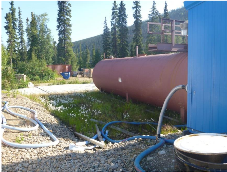
Photo 7. Fuel secondary containment system with fill material and vegetation.
