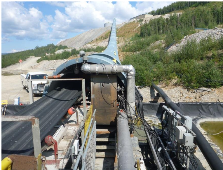
Photo 8. Former Splice House area where paste spill occurred. Plastic liner is part of new secondary containment system. Pipe coming out of blue tube is the paste line that enters into the 1690 portal.
