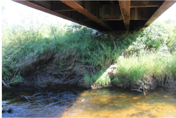
Photo 22. Gilles Creek Bridge, Abutment Scour, East Bank
