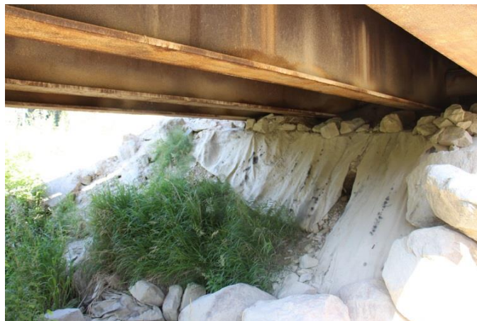
Photo 18. Shaw Creek Bridge, Degraded Scour Protection
