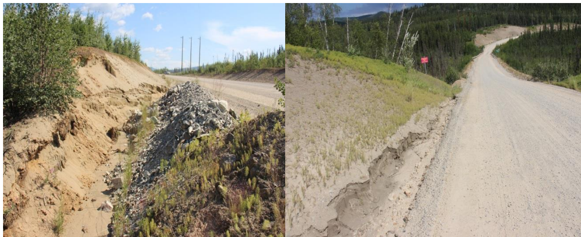
Photo 34. Erodible Soil (Sand) on Road Cut
