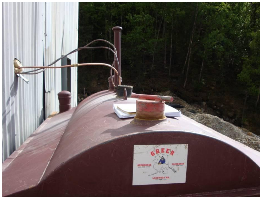
Photo 4: AST-50 showing no Access Plug to Monitor Secondary Tank Interstitial Space.
