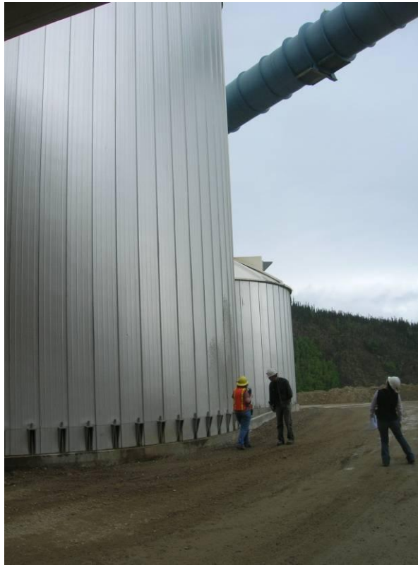
Photo 9 : CIP Tailings Storage Tank Located outside of the Paste Plant. Lack of Adequate Secondary Containment.
