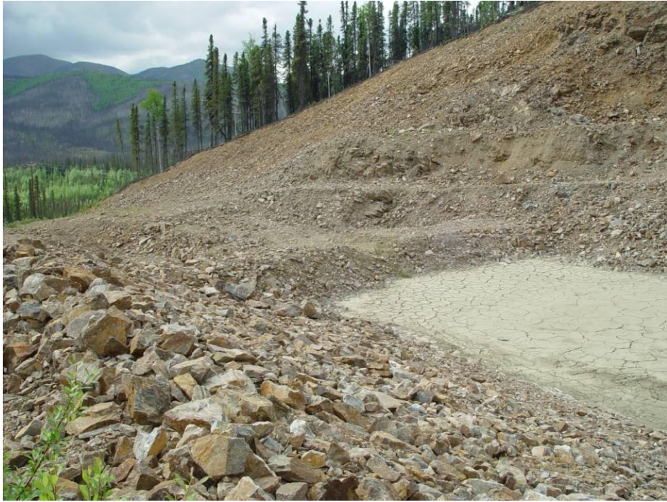
Photo 5: Sediment Accumulation in Sediment Pond in Material Site A.
