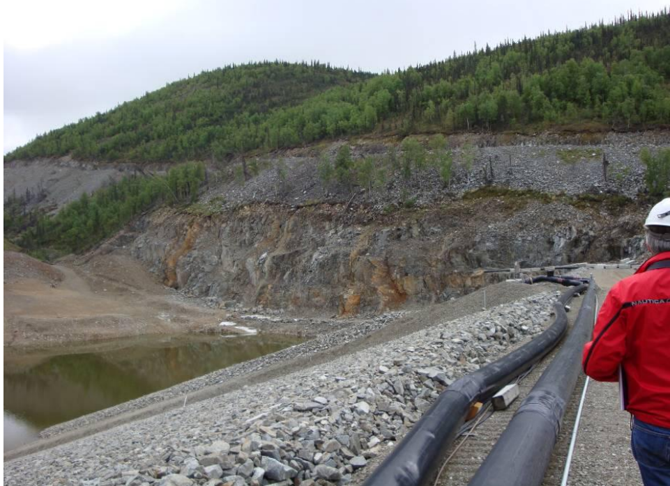
Photo 14: Upstream Side of RTP Dam with Survey Stakes to Determine Impounded Water Elevation.
