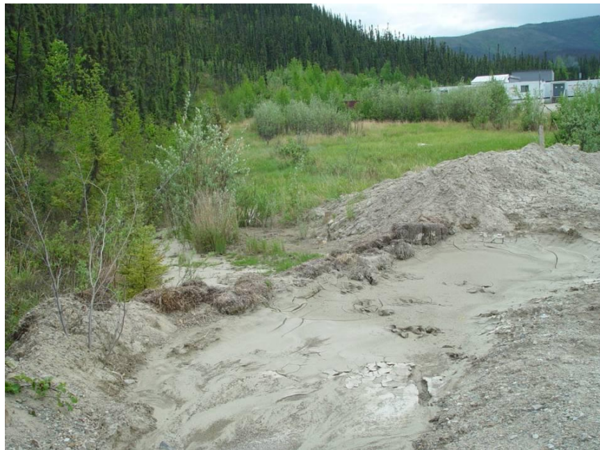
Photo 8: Sediment Accumulation Pond at the Construction Camp. Removed Sediment is Piled adjacent to Pond.
