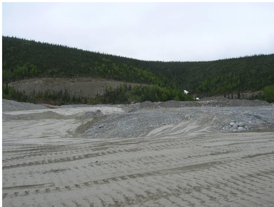
Photo 2: Rock Placement and Tailings Compaction at the Drystack Tailings Area. Mineralized Rock Entombed inside the Dry Tailings at the Drystack Tailings.
