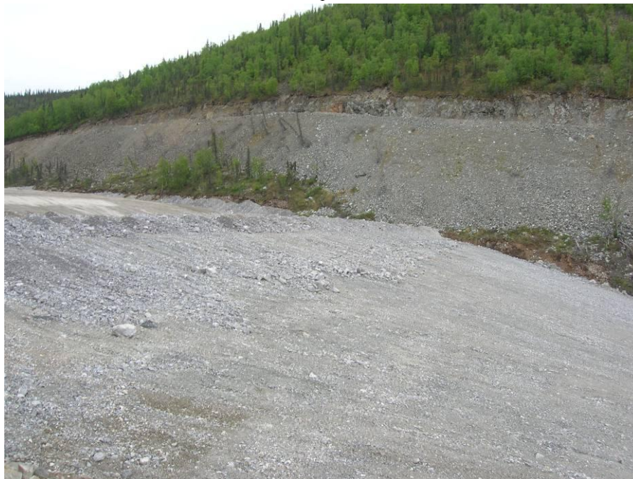
Photo 1: Upstream Shell of Dry Stack Tailings Constructed from Non-mineralized Development Rock.
