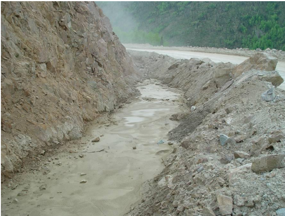
Photo 6: Sediment Buildup in Interior Road Ditch near Mill.
