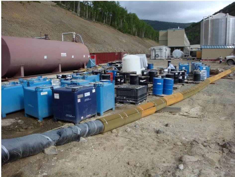
Photo 3: Secondary Containment System for Ast-1 and Portable Tanks and Drums. Note: Drums on Pallet near Front of Ast-1 are outside of Secondary Containment.
