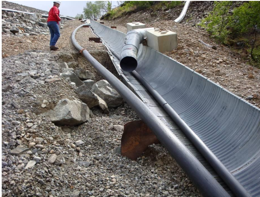
Photo 13: Erosion along RTP Dam Flume Spillway from Diversion Ditches Discharge Outlet.
