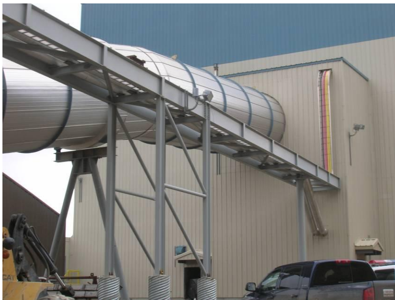
Photo 10: Overhead Pipelines Delivering Tailings from the Cyanide Destruction System in the Mill to the CIP Tailings Storage Tank. Lack of Secondary Containment.
