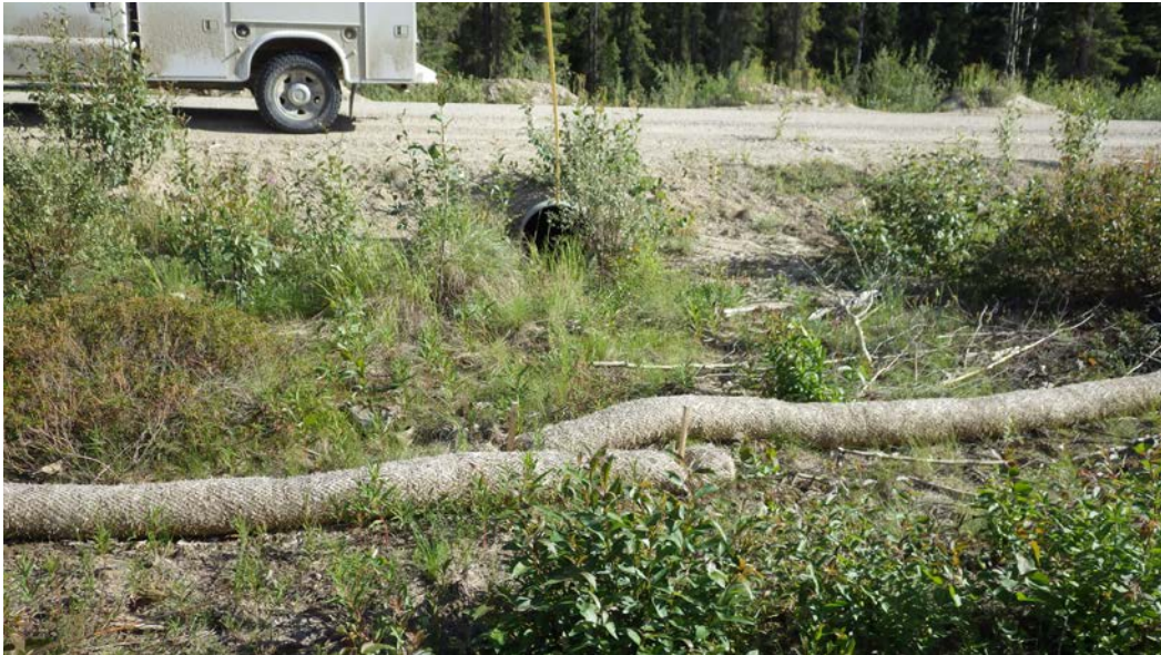
Photo 2: Erosion control under transmission line along Pogo Access Road
