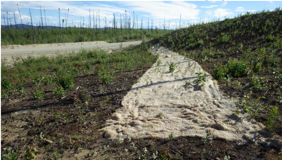
Photo 1: Erosion control under transmission line along Pogo Access Road
