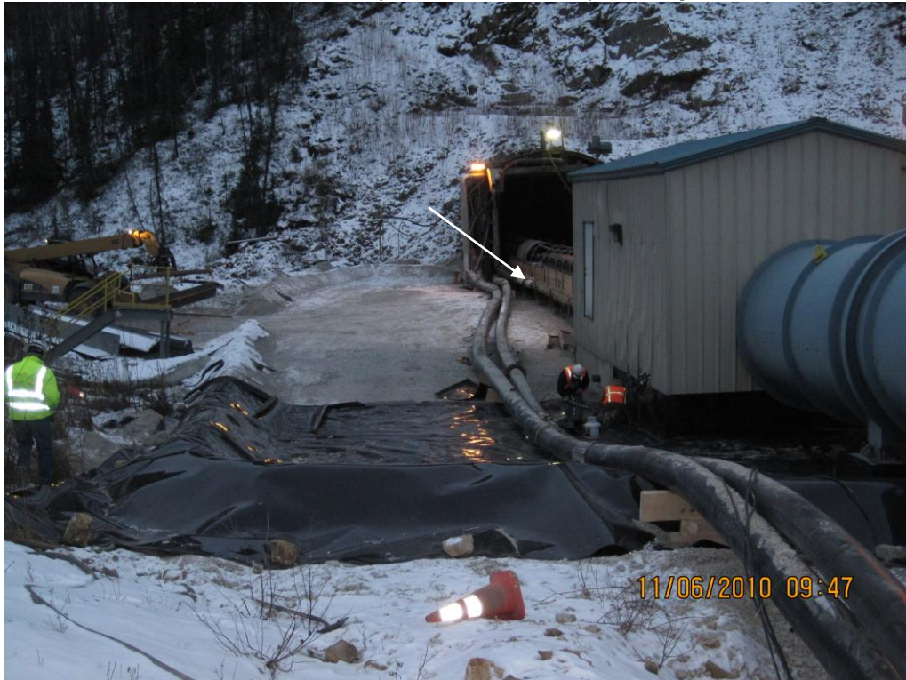
Photo B - 1690 Portal Secondary Containment (arrow points to Paste Line)
