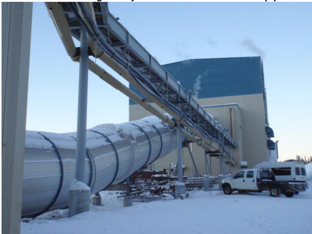
Photo C - CIP Tailings Slurry and Backfill Dilution Water pipelines
