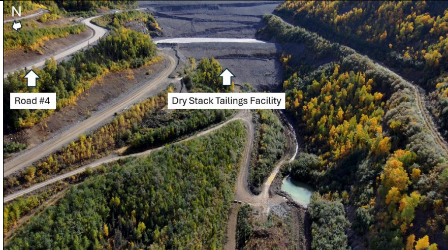
Photo 3: Another view of the DSTF shells from above the RST. Note the Stilling Basin center bottom right of the photo.
