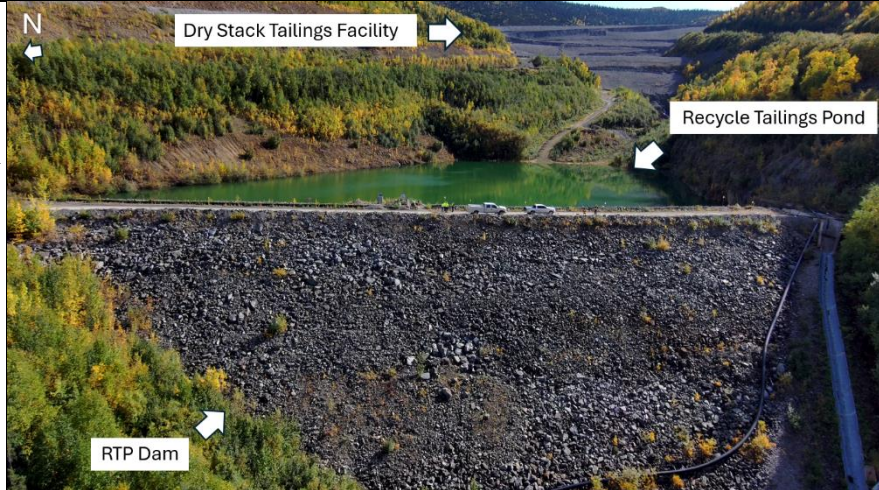
Photo 5: Another view up valley of the RTP and RTP Dam. Shells of the DSTF in the background. Note vehicles for scale on the top of the dam and spillway on the right side of the photo.
