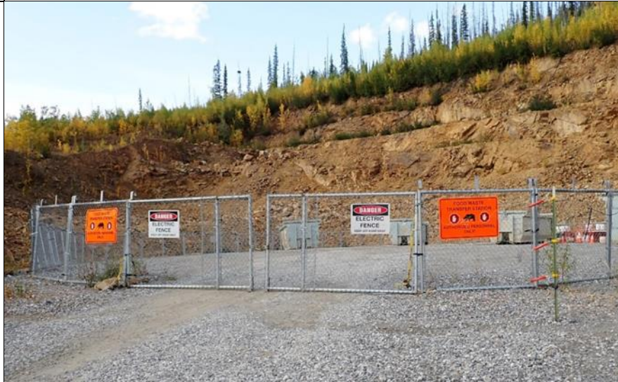
Photo 16: Food Waste Storage and Kinetic Testing Area. Fence is electrified to keep wildlife from entering the area.
