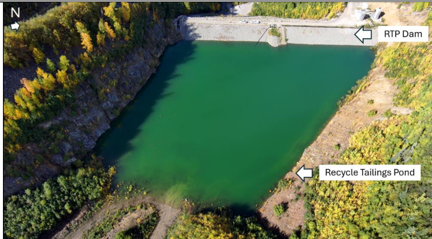
Photo 6: View of RTP Dam and water level. Note RTP Head Tanks in the upper right corner.
