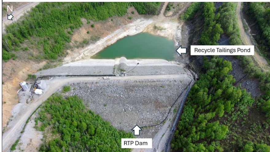
Photo 6: Another view of the RTP and RTP Dam. Note vehicles for scale on the top of the dam, RTP Head Tanks to the left and spillway on the right.
