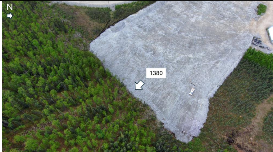
Photo 10: Another view of the 1380 Area access pad where it meets the slope of the hill. Note truck for scale.
