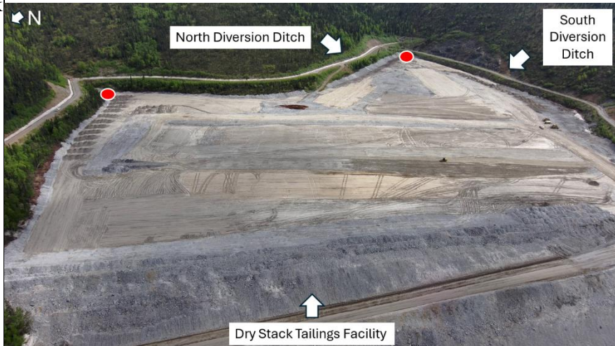
Photo 2: Another view of the DSTF. Red dots mark areas of Flow Through Drains.
