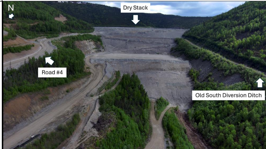
Photo 4: Another view of the DSTF tiered development and shells from above the RST.
