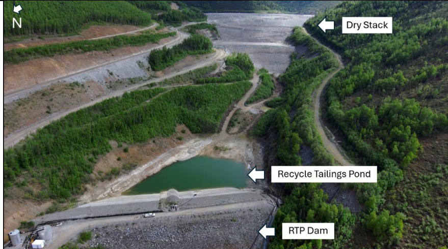
Photo 5: DSTF, RTP, and RTP Dam. Note the low water level behind RTP.
