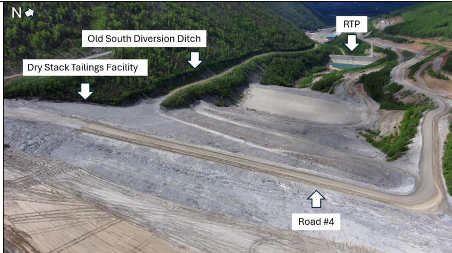
Photo 3: A down valley view of the DSTF. Note the levels of tiered development and shells on the front leading to the toe.
