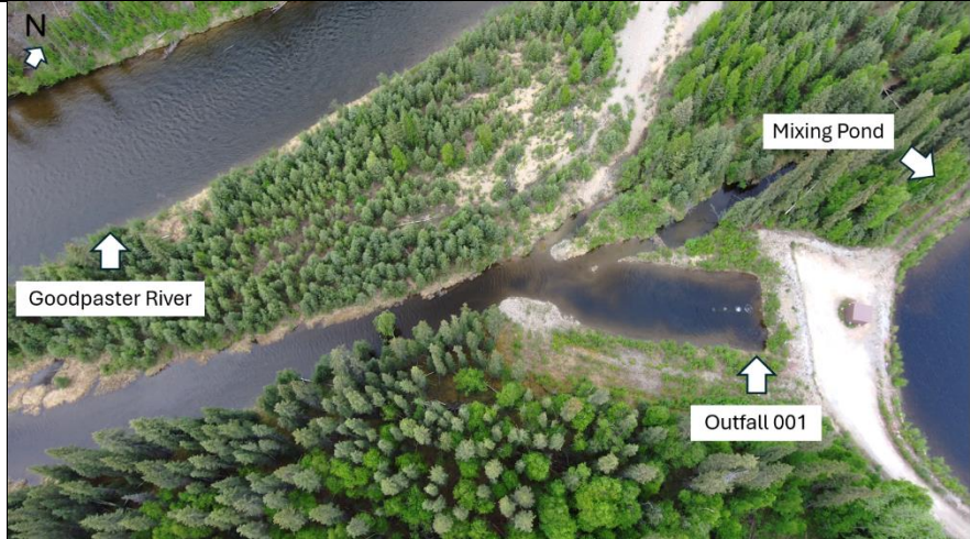
Photo 13: Location of Outfall 001 in relation to the Mixing Pond and Goodpaster River.
