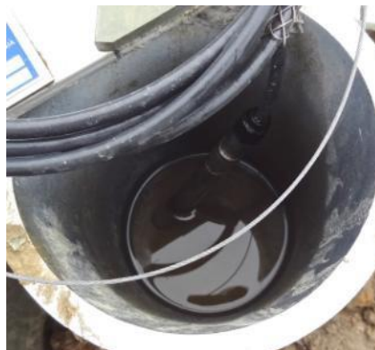
Photo C-4: PT Installed in Flume Stilling Well
