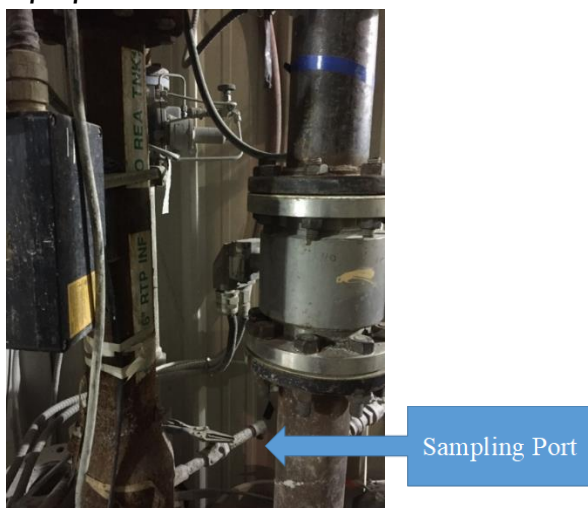
Figure 7. WTP-FEED1 sample port at MWTP#3 RTP head tank water influent pipe
