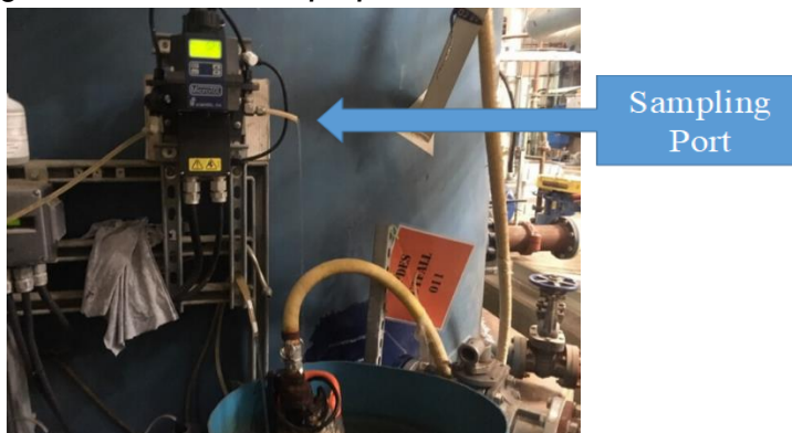
Figure 5. OUTFALL011 sample port at turbidimeter
