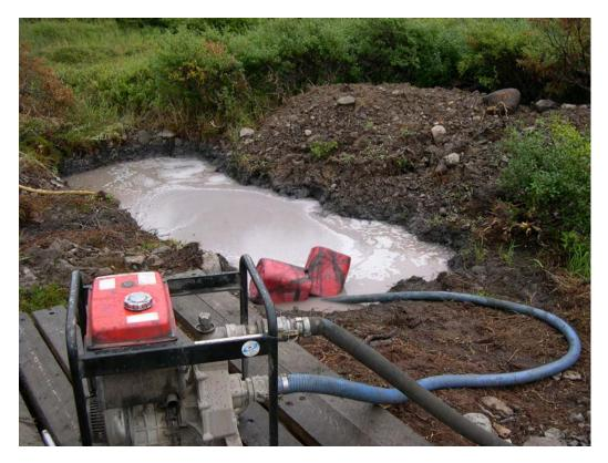
Figure 4. Settling pond at drill site.
