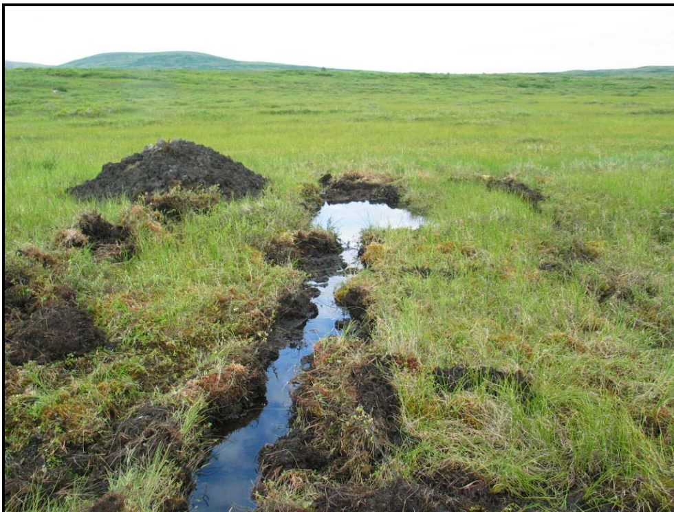
Photo #12. Drainage ditch and sump at new drill site.
