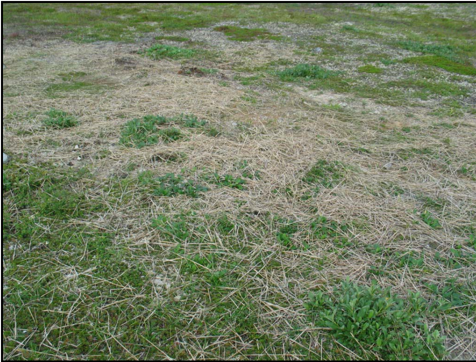
Photo #39. Reclamation at DDH 7364. Site has been treated with straw to prevent erosion, and seeded with grass. Note new vegetation.
