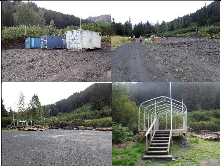
Photo 8-11: Views of the Laydown Yard. Cleared, clean, and prepared for winter.
