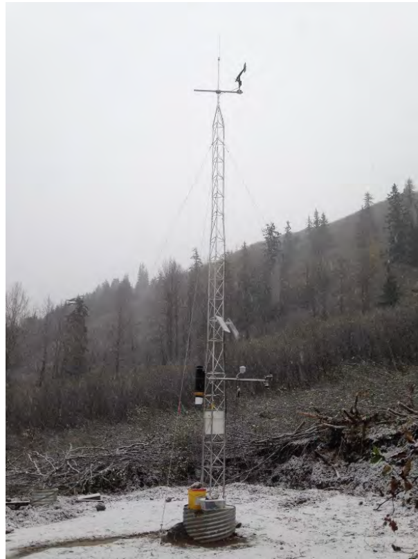
Plate 6.1: Meteorological Station (facing east)
