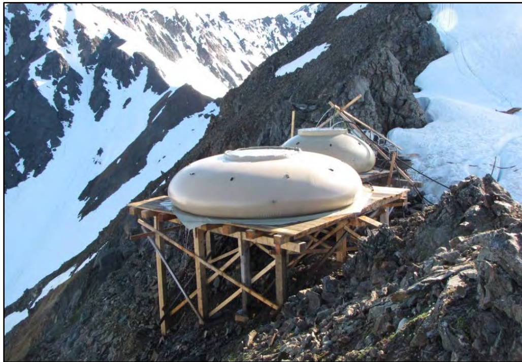
Plate 2.1: Typical Water System Setup showing collapsible bladders/platform/hose Line
