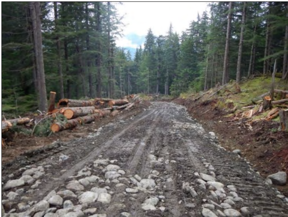
Plate 2.10: Construction of 2014 Exploration Access Road
