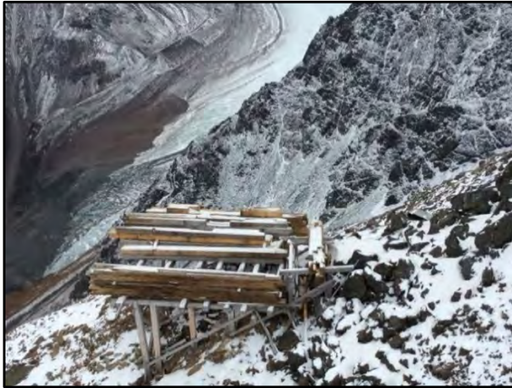
Plate 3.1: Removal of decking material
