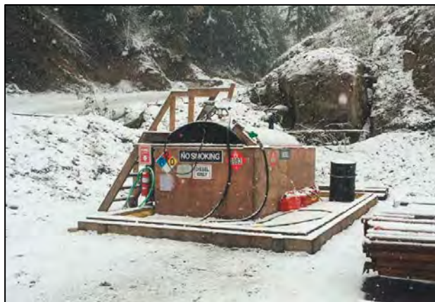
Plate 2.5: Fuel tank and containment system for a 3,000 gallon diesel fuel storage tank with secondary containment capacity of 3,300 gallons at Big Nugget Camp; a similar design would be employed for storage tanks at the proposed equipment laydown site.
