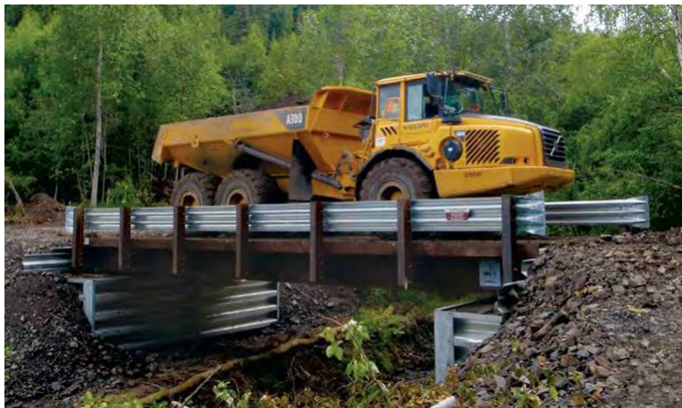
Photo 2-2. Example of Prefabricated, Modular Steel Vehicle Bridge
