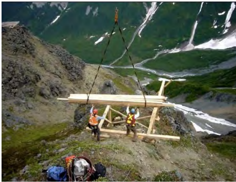
Photo 2-3. Slinging Decking Material for Drill Pad Construction
