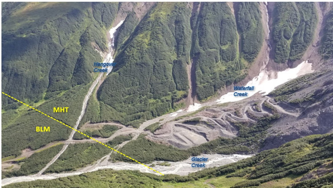
Photo 1 Aerial photo, looking SE, showing land clearing associated with Phase I & II Plan of Operations (on MHT Lands) July 31, 2019
