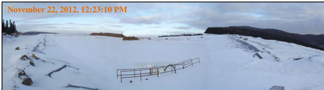
Photograph 4- FTDS Retention Pond
