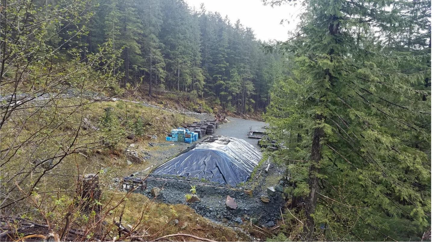
Fully lined and covered low-grade PAG ore pile
