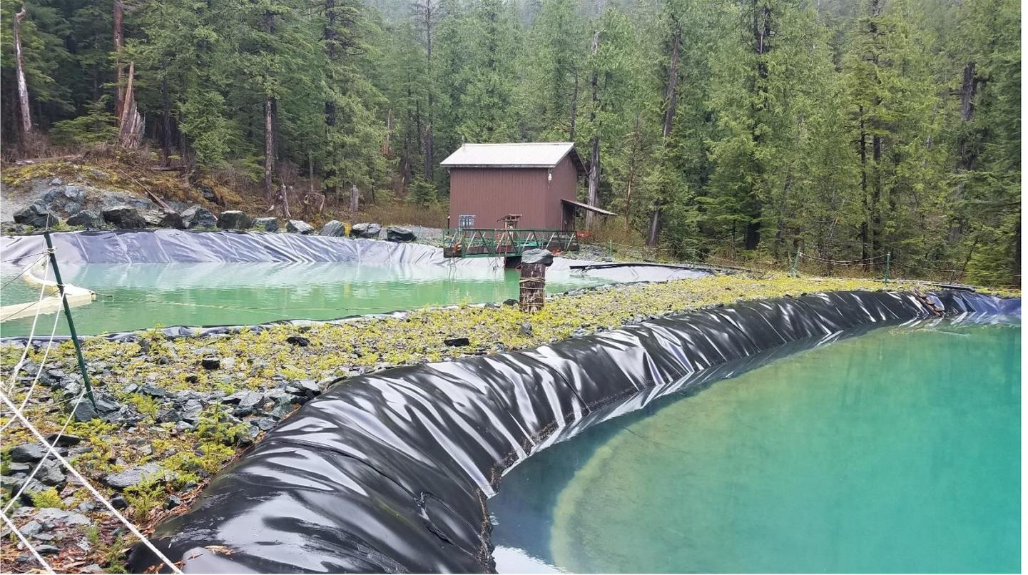
Settling ponds with water treatment facility at back
