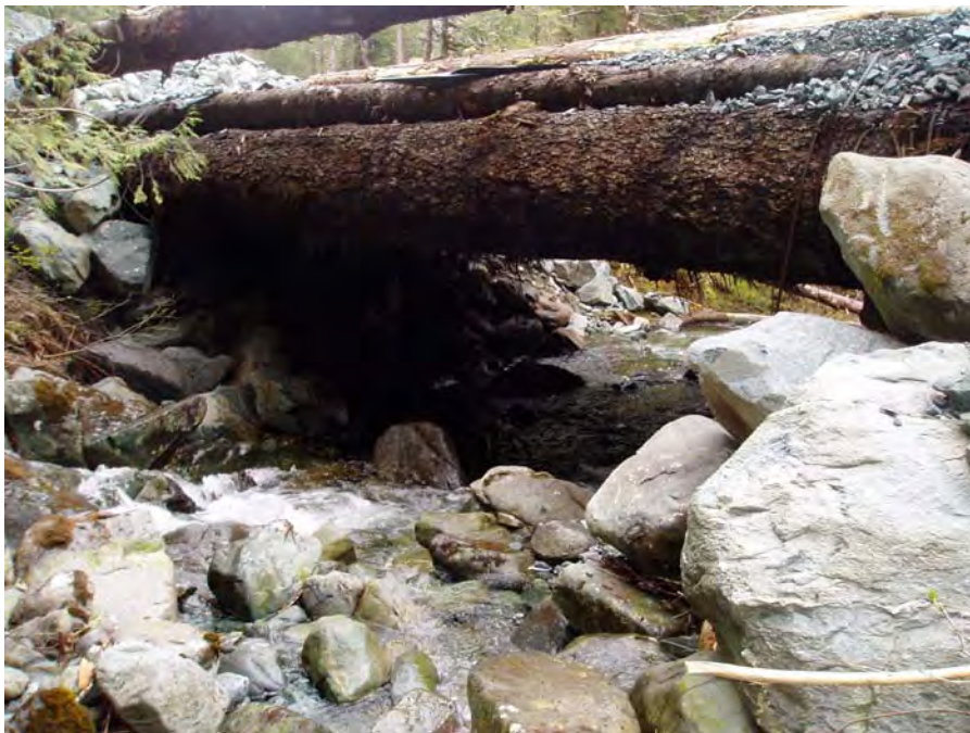
Photo 31. Surface water monitoring station WQ7, Camp Creek upstream location (looking downstream; April 2008).
