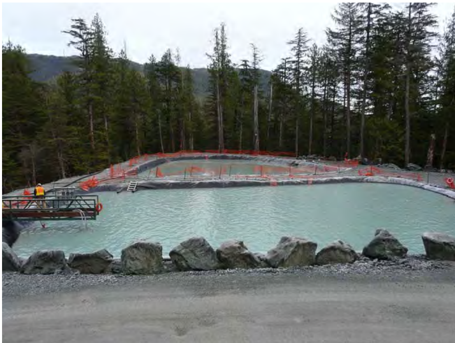
Photo 10. Completed sediment ponds (2009).
