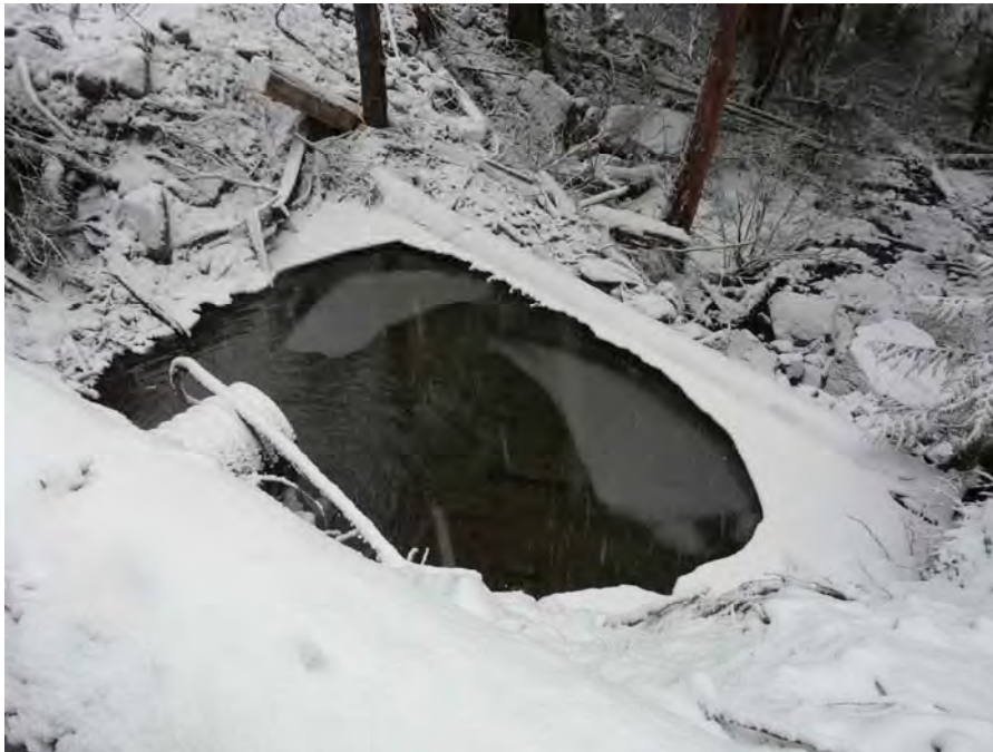
Photo 6. Culvert and sump near sediment ponds.
