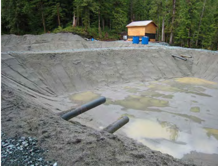
Photo 7. Sediment pond construction, including sand bedding layer (water treatment plant in background).
