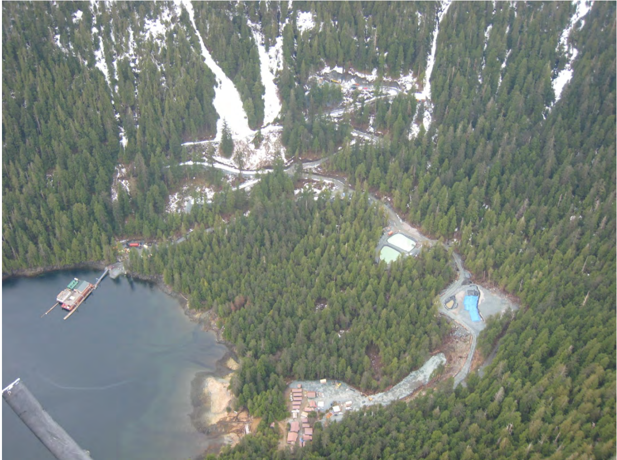
Photo 1. Aerial view of site, looking southwest (March 2008).
