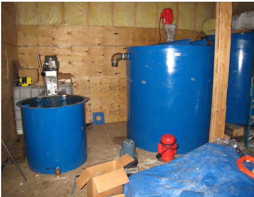
Photo 12. Partially completed water treatment facility, showing treatment tanks and mixers.
