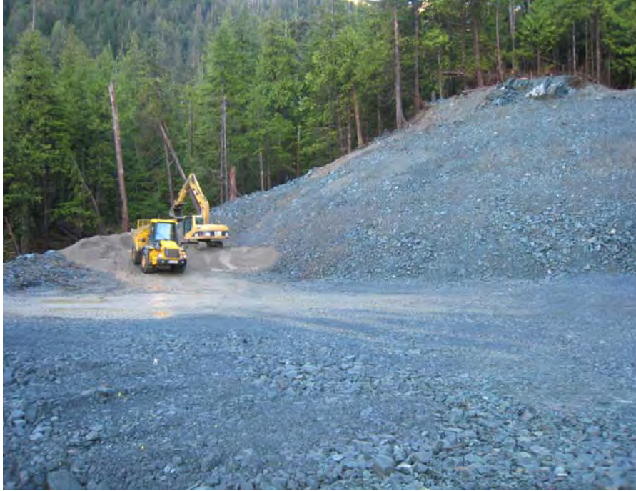
Photo 15. Crushed rock base of PAG site prior to compaction, placement of sand layer, and liner installation (November 2007).
