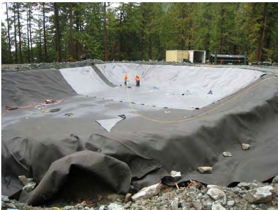
Photo 8. Sediment pond construction, showing geotextile placement, anchor trench, and HDPE liner.
