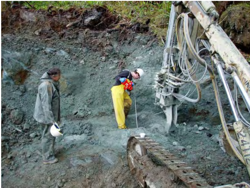
Photo 44. Construction of groundwater monitoring well MW8 (June 2007).
