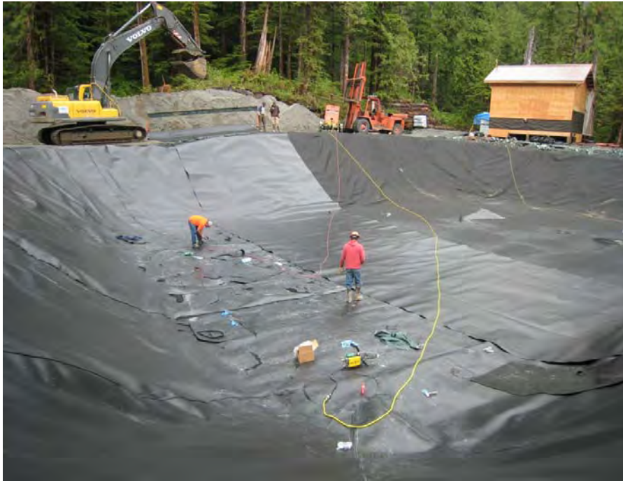
Photo 9. Sediment pond construction, showing HDPE liner installation.
