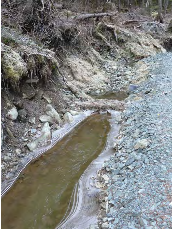
Photo 4. Roadside ditch including culvert and straw bale sediment trap.
