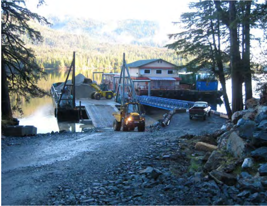
Photo 22. Barge ramp, float dock, and floating barge camp.
