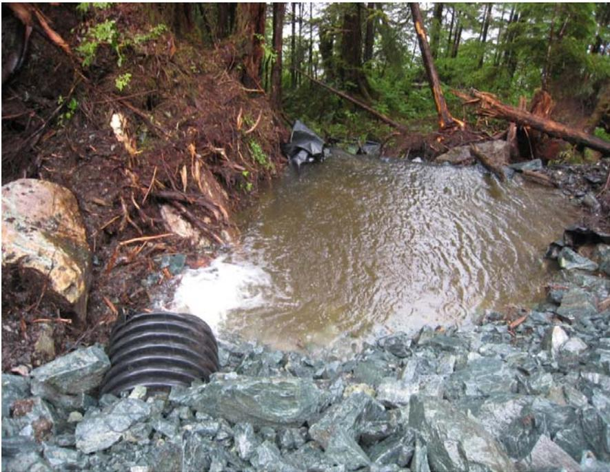
Photo 4. Sediment trap located along road down slope of NAG waste rock site. Photo taken during period of heavy rainfall.
