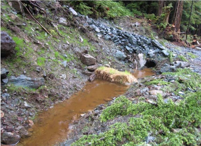
Photo 2. Roadside ditch including culvert and straw bale sediment trap. Note freshly seeded road cut/slope.
