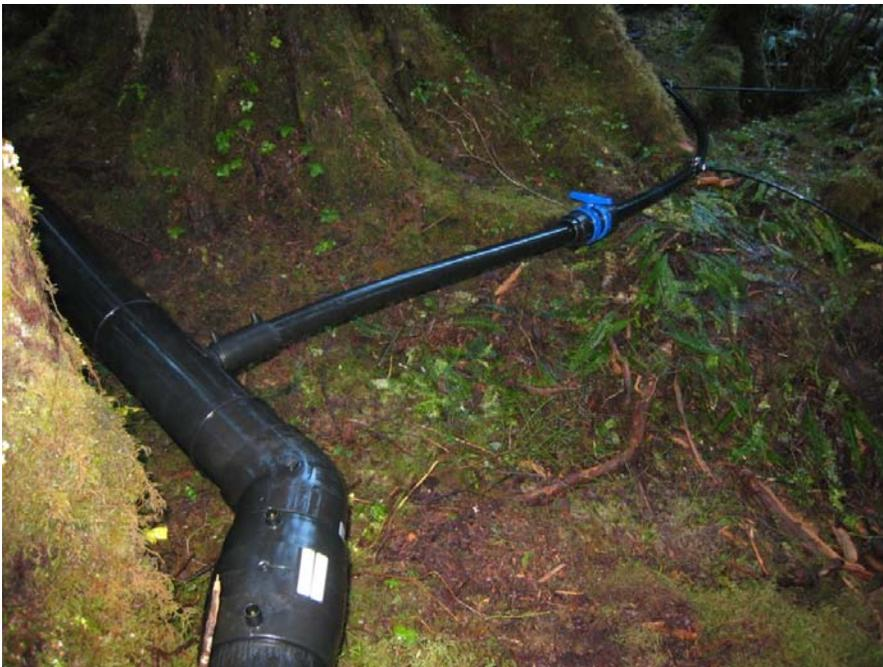
Photo 10. Land Application Area, distribution system with 6-in. main line connecting to 2-in. pipe that services drip emitter lines for a single land application zone.
