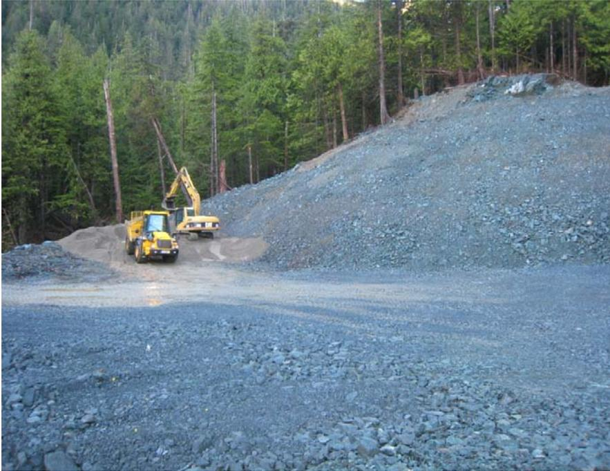
Photo 11. Crushed rock base of PAG site prior to compaction, placement of sand layer and liner installation (November 2007). Construction not complete at year end.
