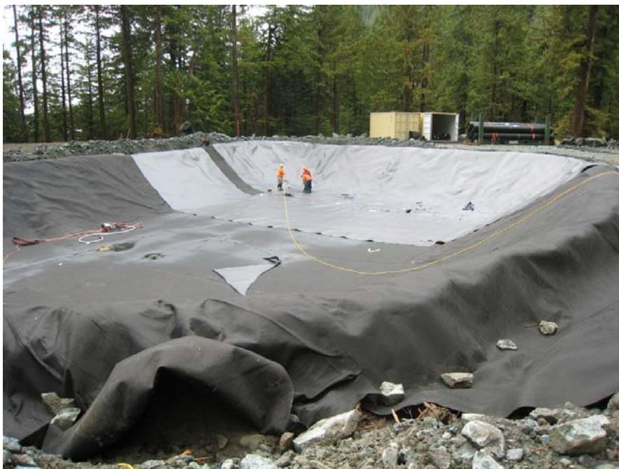
Photo 6. Sediment pond construction, showing geotextile placement, anchor trench, and HDPE liner.
