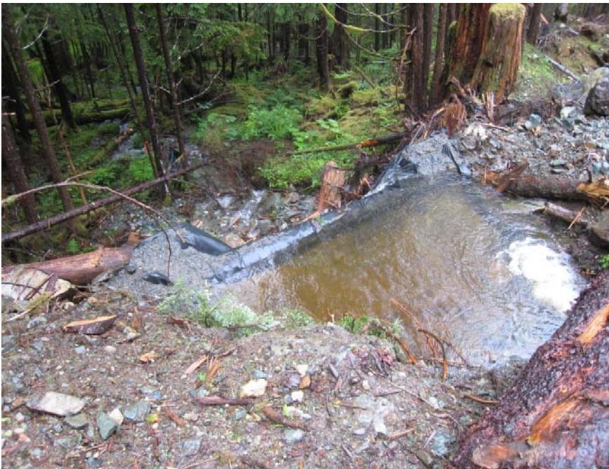
Photo 3. Sediment trap located along road down slope of NAG waste rock site. Photo taken during period of heavy rainfall.
