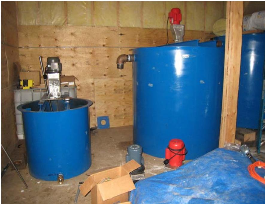
Photo 8. Partially completed water treatment facility, showing treatment tanks and mixers.
