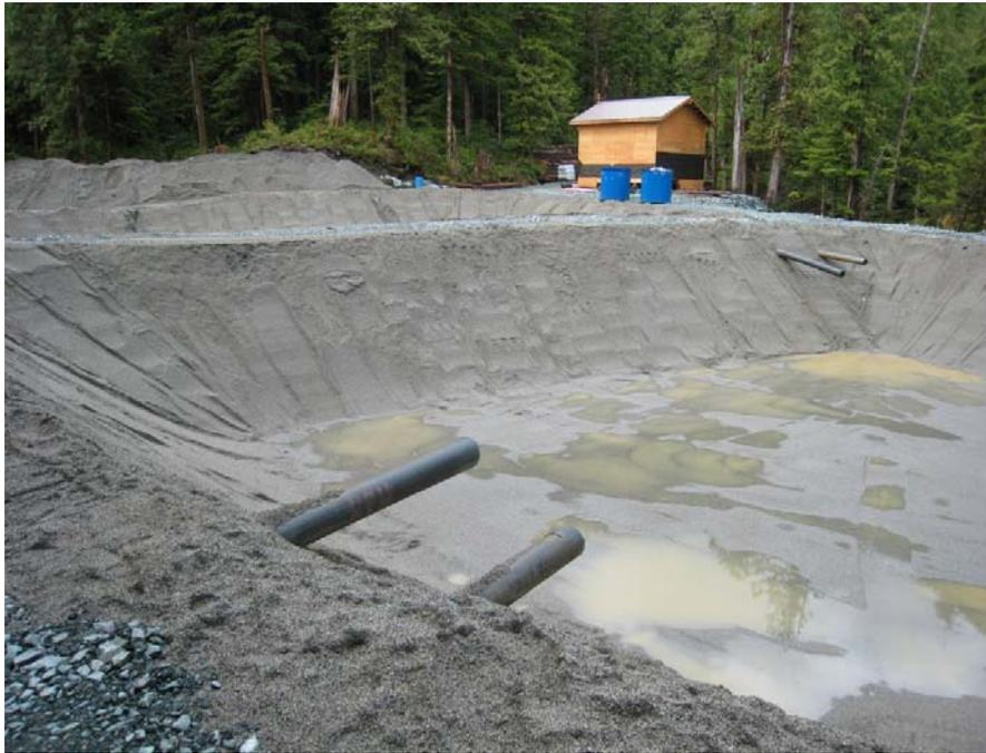
Photo 5. Sediment pond construction, including sand bedding layer (water treatment plant in background).
