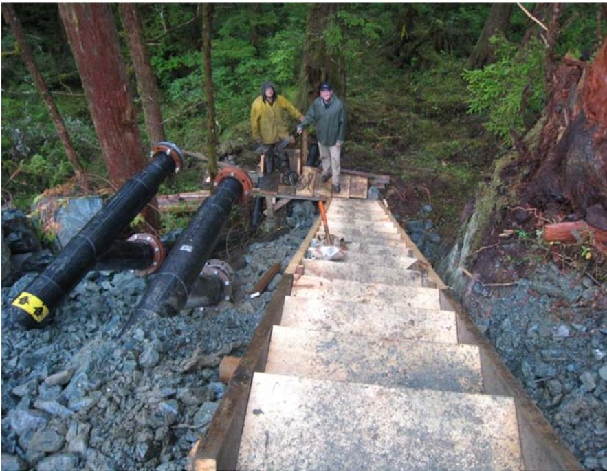
Photo 9. HDPE pipes exiting water treatment facility/sediment ponds and leading to Land Application Area.
