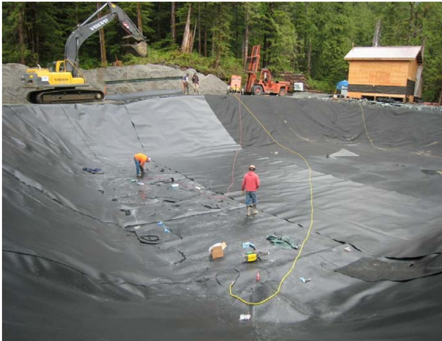
Photo 7. Sediment pond construction, showing HDPE liner installation.
