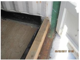
Photo 12. A TTF water treatment plant storage container with secondary containment.
