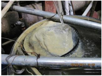
Photo 5. A rock used for monitoring white material accumulation at the Comet water treatment plant.
