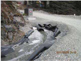
Photo 21. Stormwater runoff in the drainage ditch is mostly frozen over image 1 of 2.
