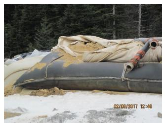
Photo 10. Dewatering bag is torn and will be replaced when dredging begins at Comet.
