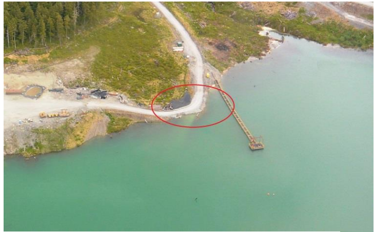
Figure 4 Filled road bed area.
