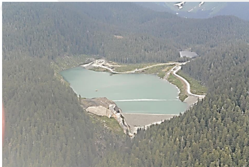
Figure 1 Aerial view of the Tailings Treatment Facility.
