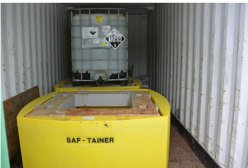
Figure 7 Internal, individual secondary containment for muriatic acid.
