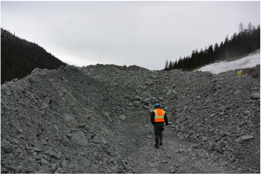
Figure 9 The pile is beginning to be pushed south toward the camp.
