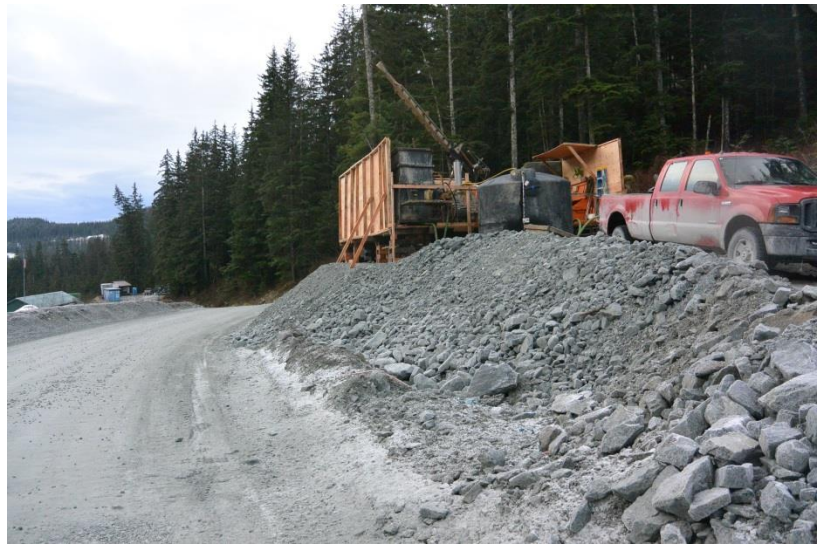
Figure 2 Surface exploration drill pad.
