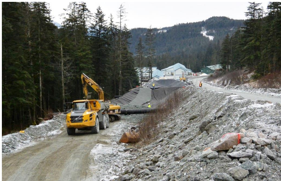
Figure 10 Construction of two new storm water runoff ponds was nearly complete.
