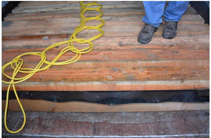
Figure 6 Internal secondary containment designed and constructed by Pete Strow. A very robust design.
